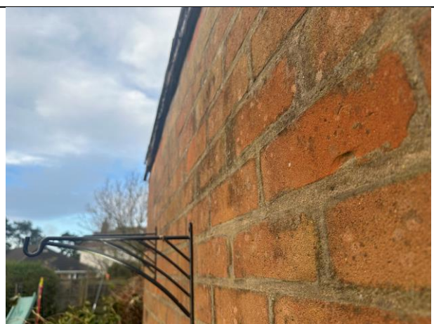
Photo 4 Sealed fascia at single storey section
