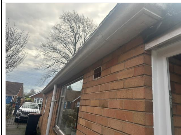
Photo 3 Sealed finlock gutter
