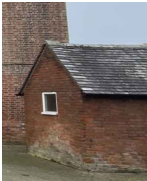
Existing Brick Shed to be removed
