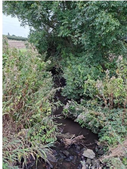
Figure 3: WC2 – Overview (within channel)
