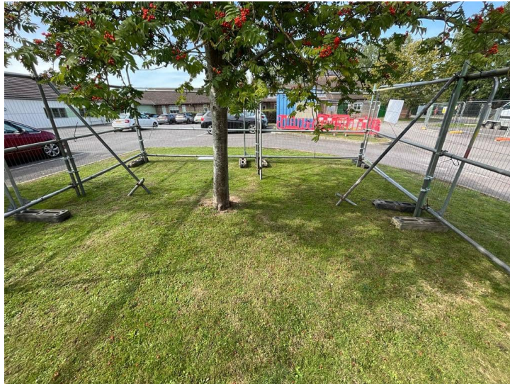
Photograph 5 (Onsite example of tree protection barrier installation)
