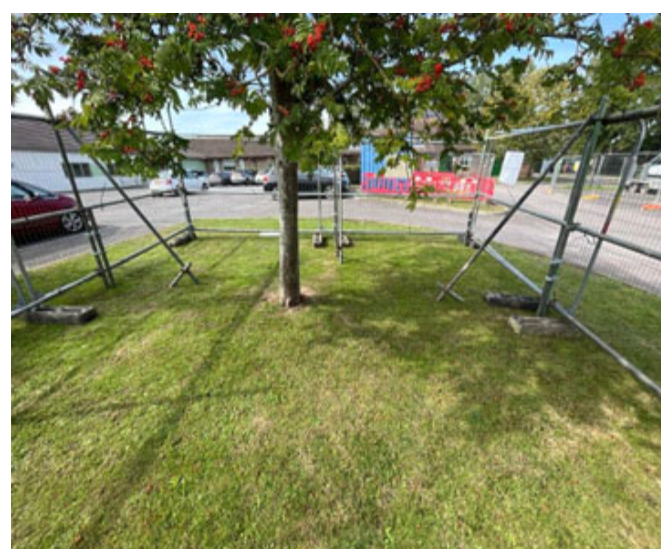
Onsite example of tree protection barrier installation
