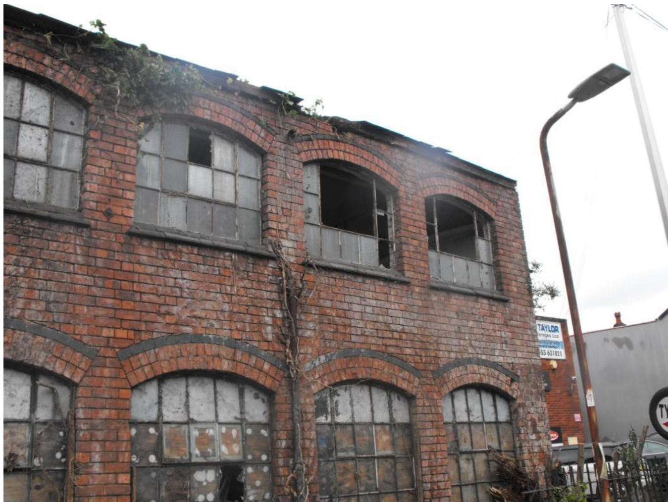
Building 1 external: all gaps in brickwork at ground level inspected via a ladder and endoscope, druid Street elevation
