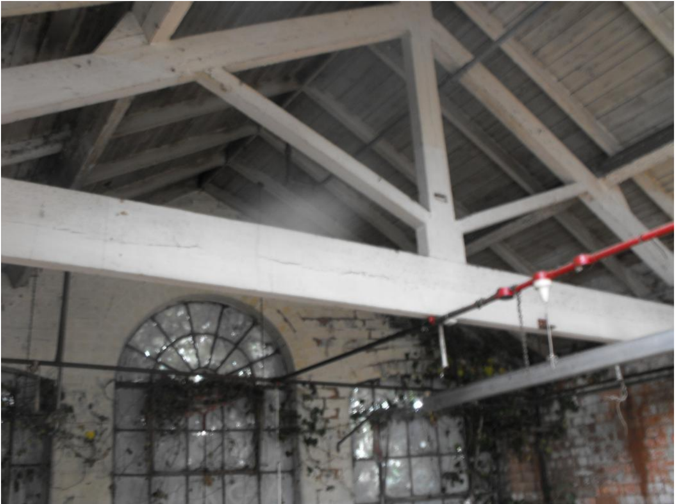
Building 1 upper ection
