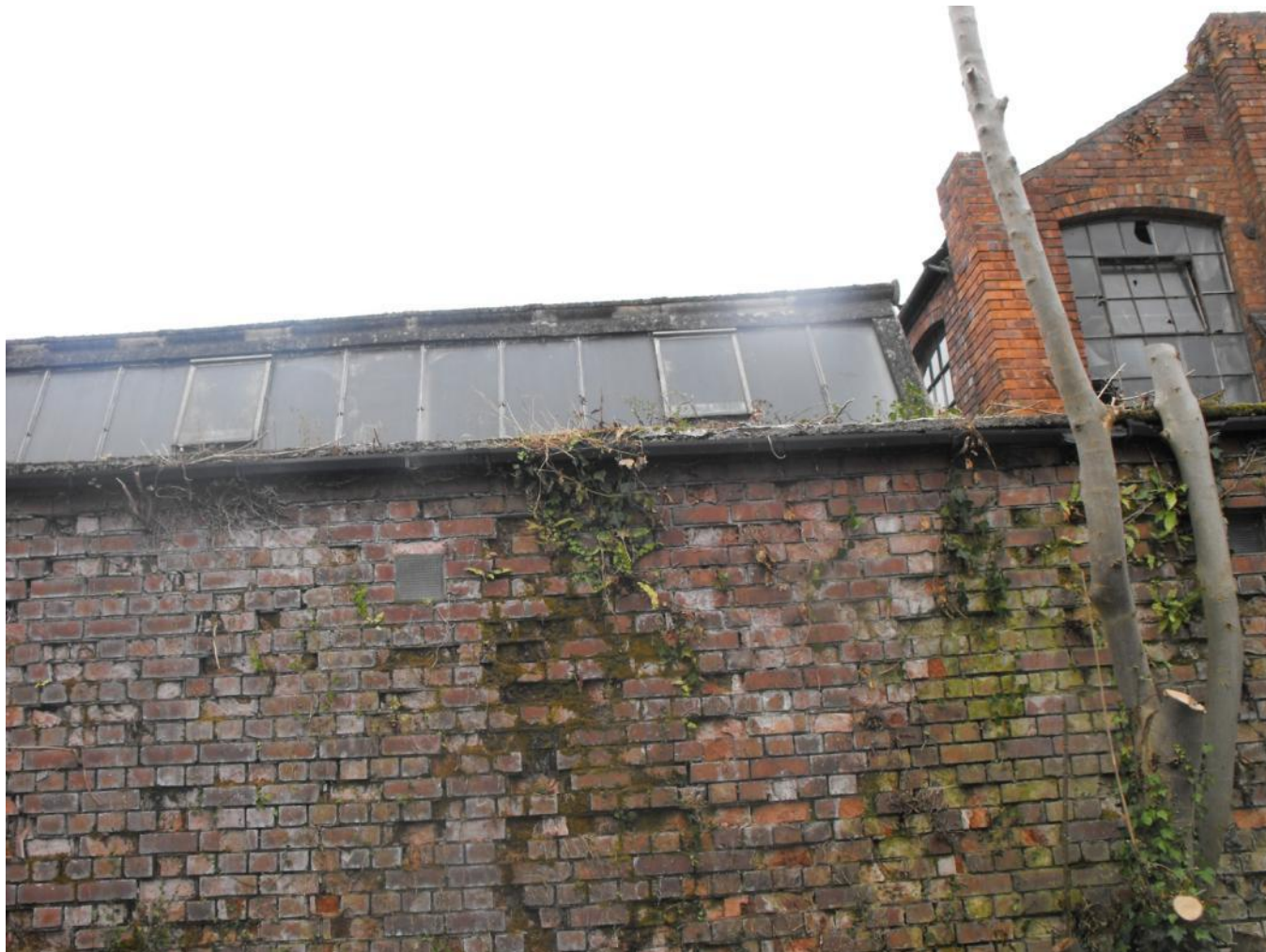
Rear of building 2 (left) and Building 1 (right)
