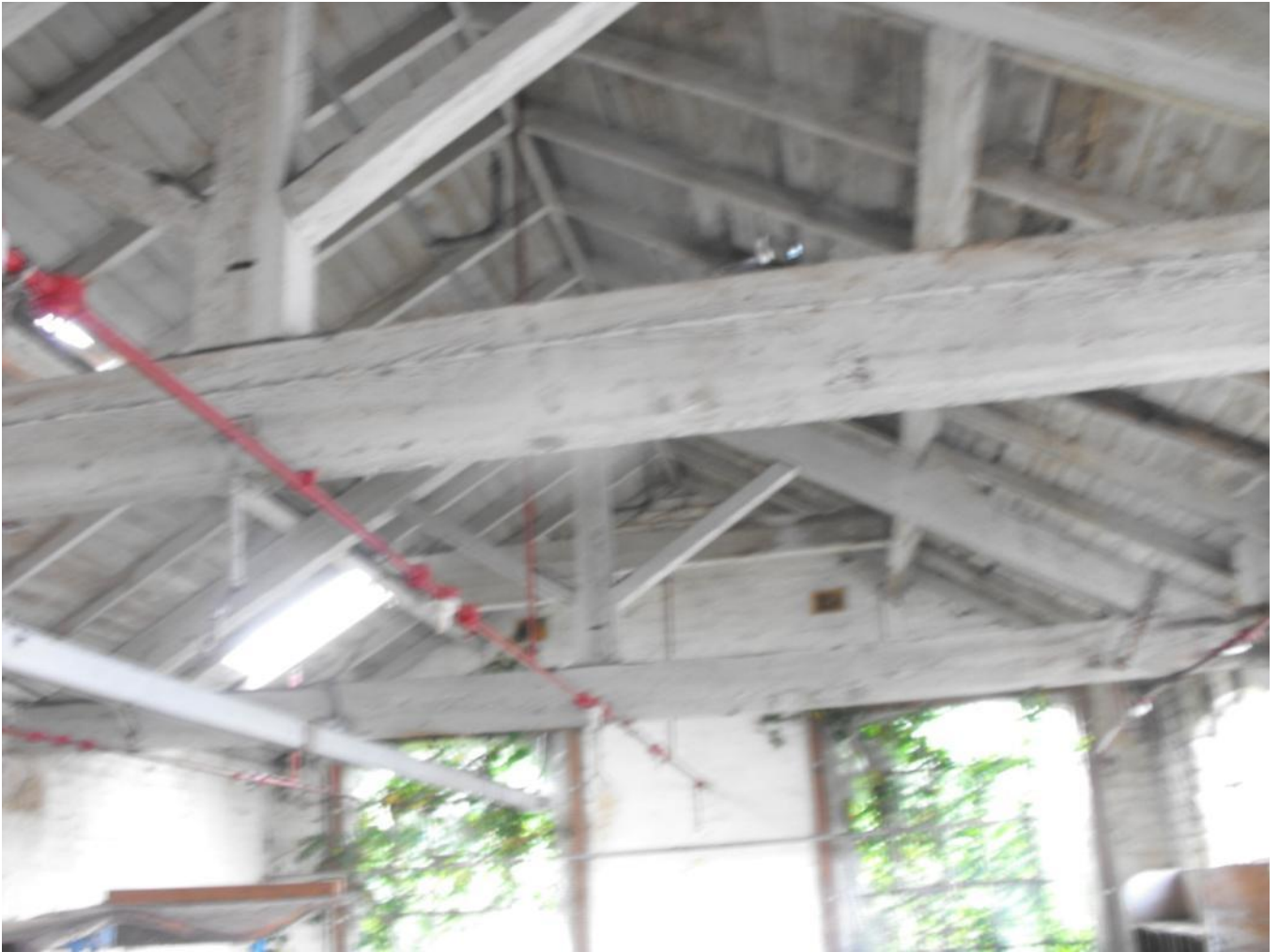
Building 1 upper section
