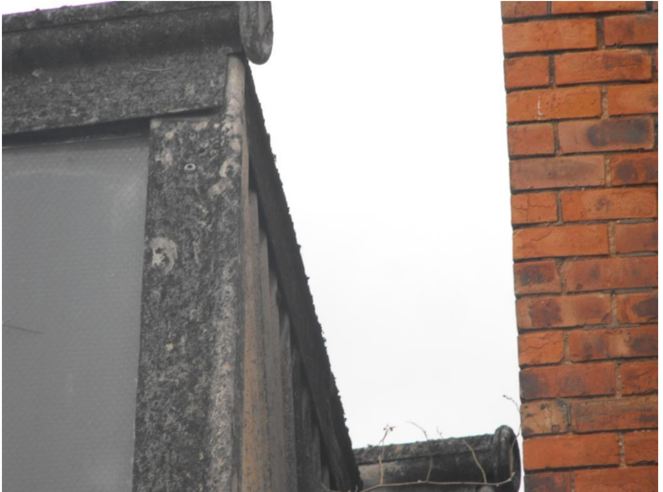
Building 2 roof detail
