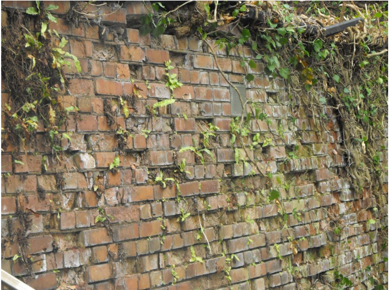
Building 2 Rear wall, gaps inspected with endoscope
