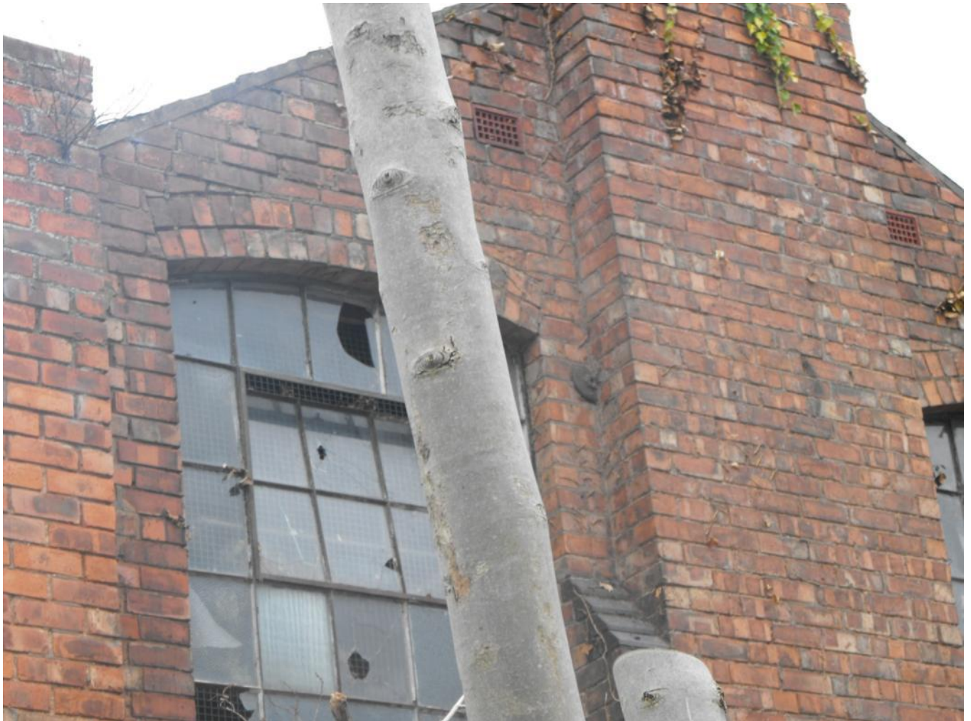
Building 1: External, rear image
