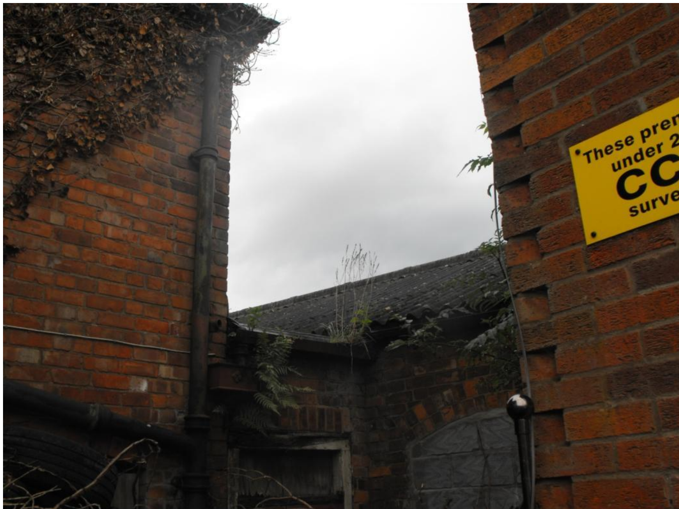
Detail of roof Building 2
