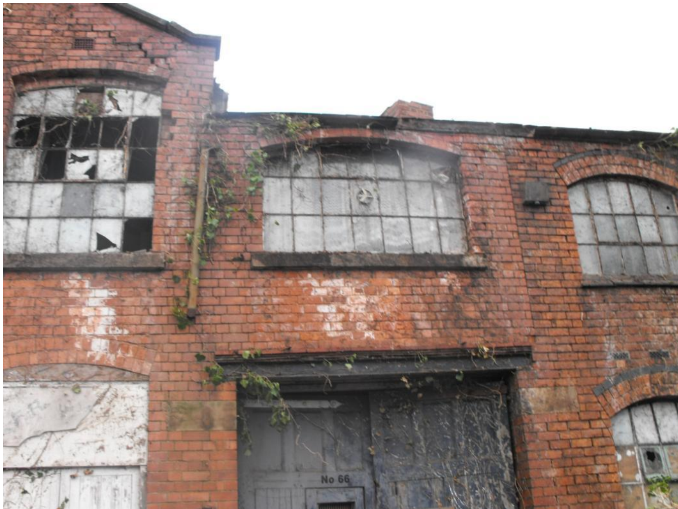
Building 1 external: all gaps in brickwork at ground level inspected via a ladder and endoscope
