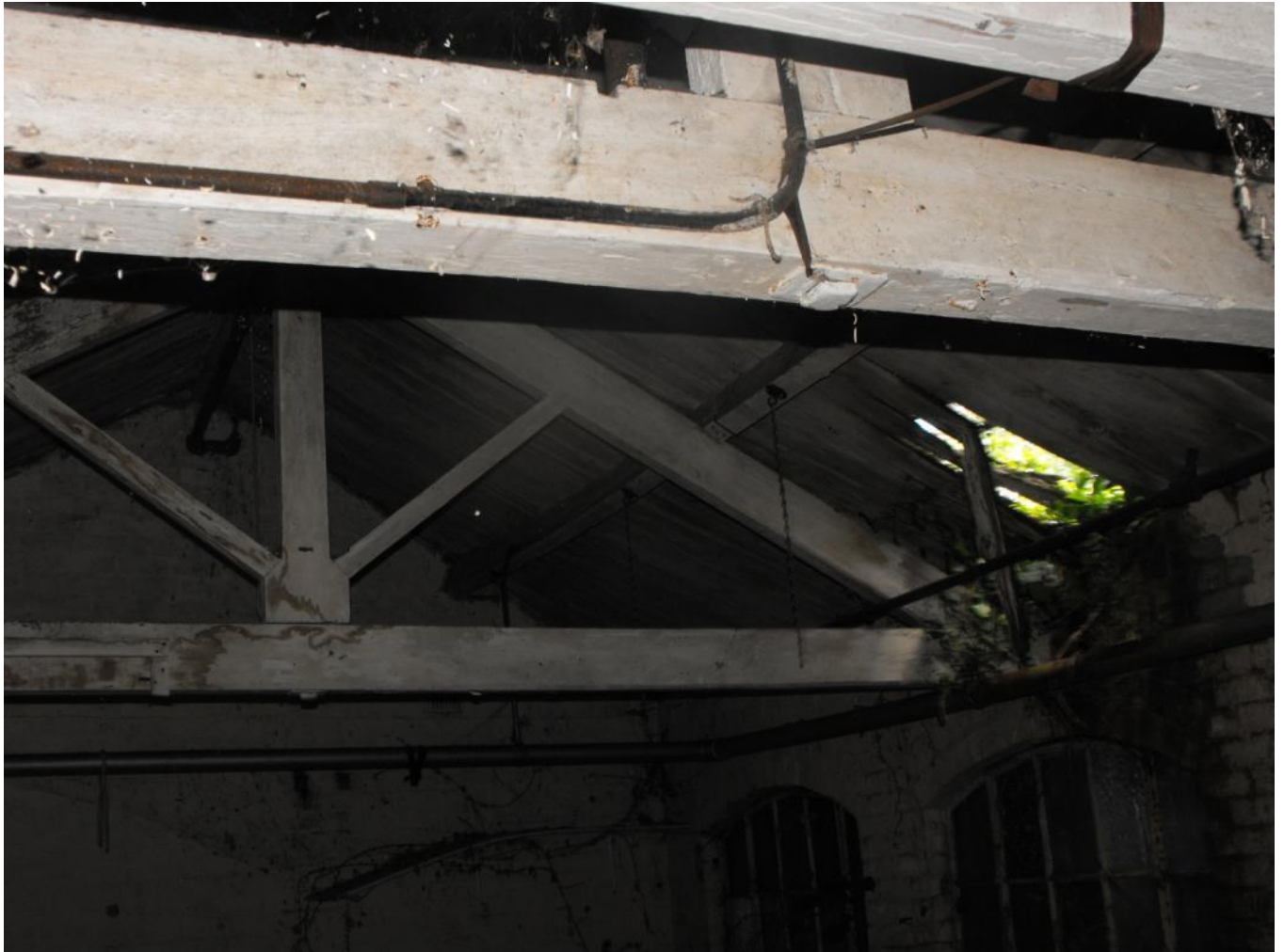
Building 1 upper section
