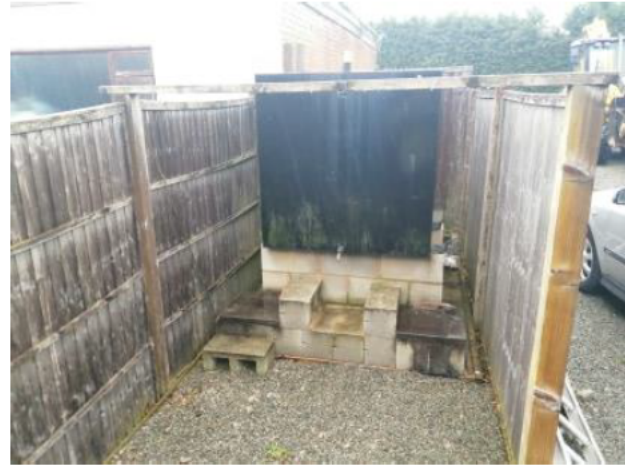
Photo 4: Oil AST (Front of site) / Facing NE
