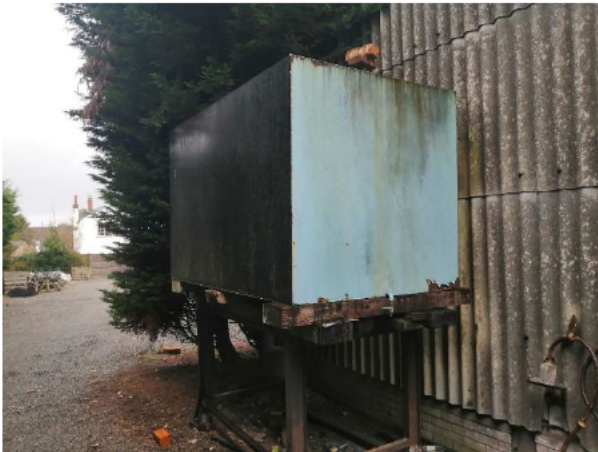
Photo 1: AST (Rear of site) / Facing NW
