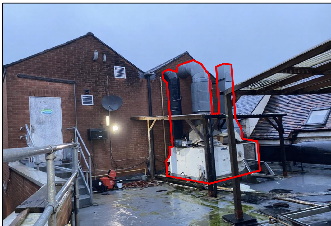
Figure 4: Mechanical plant to be removed in the first-floor rooftop garden area
