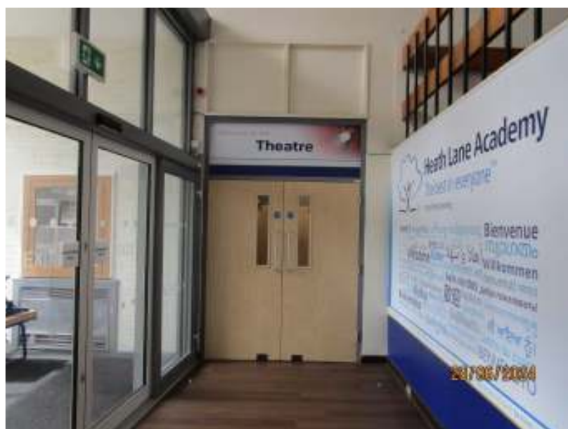
Image 08: Existing internal door to reception area to be provided with access control.
