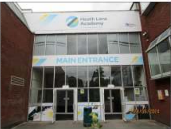
Image 01: Existing school entrance screen & signage to be replaced.
