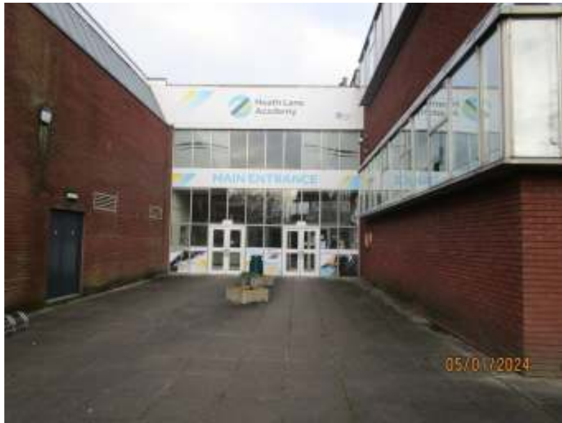
Image 01: Main school entrance showing the existing glazed screen with entrance and exit doors.
