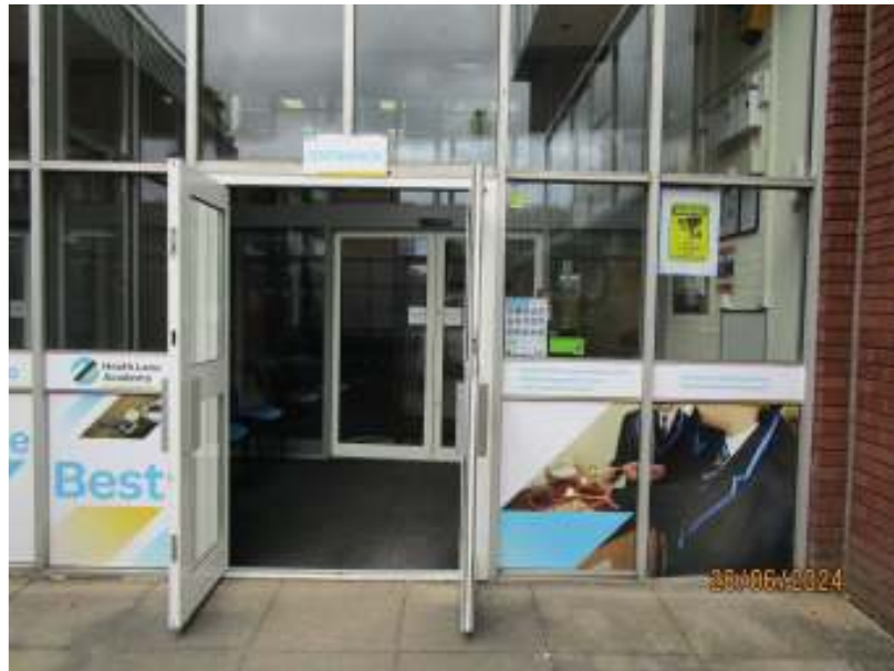
Image 03: Existing manually operated entrance doors to be replaced with new fully automatic sliding doors.
