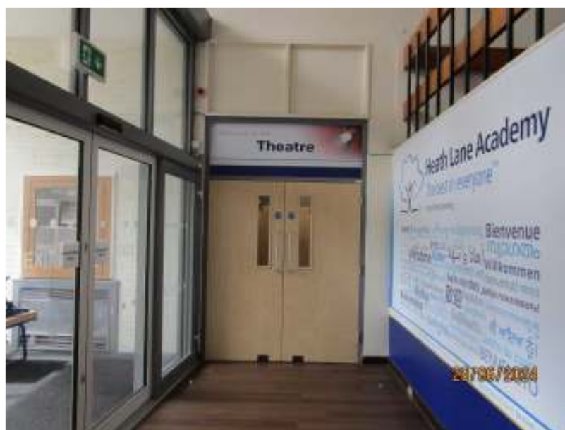
Image 08: Existing internal door to reception area to be provided with access control.
