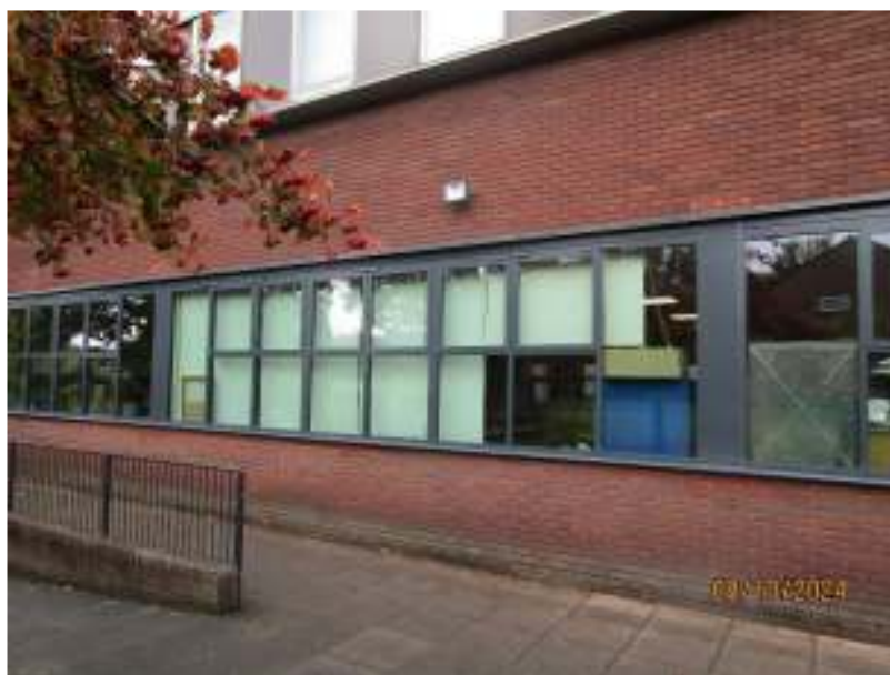
Image 07: Typical image showing the new windows installed to the ground floor of the main block. The proposed entrance screen will match the colour and finish of the new windows, RAL 7016 Anthracite Grey.
