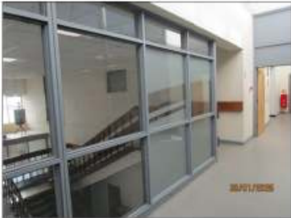
Image 02: Proposed location of automatic powered sliding door to first floor level at top of stairs. Sliding door to open back in front of the existing timber glazed screen.
