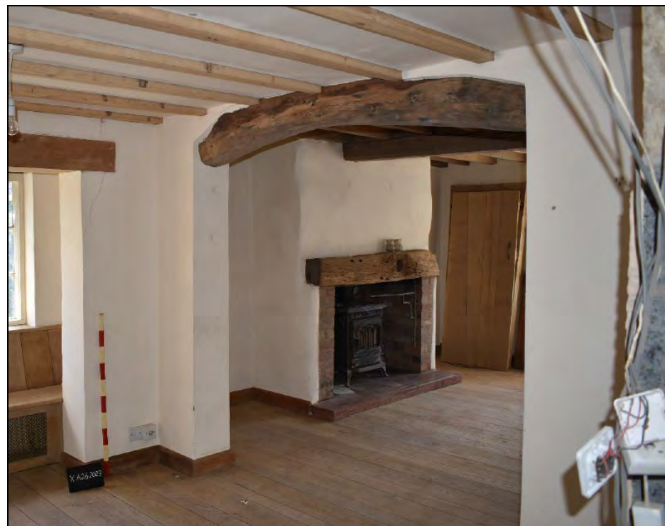
Plate 21: GF04 looking SSE into GF12 (1.0m scale)
