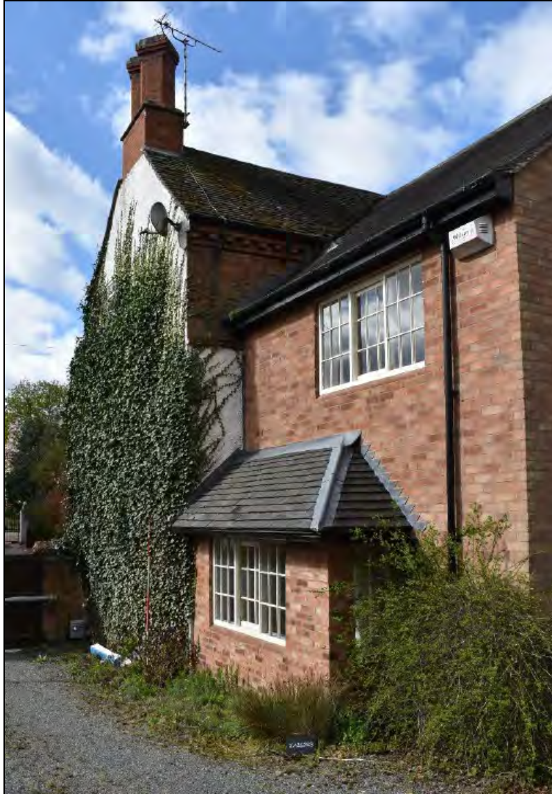
Plate 6: East elevation looking SSW (2.0m scale)
