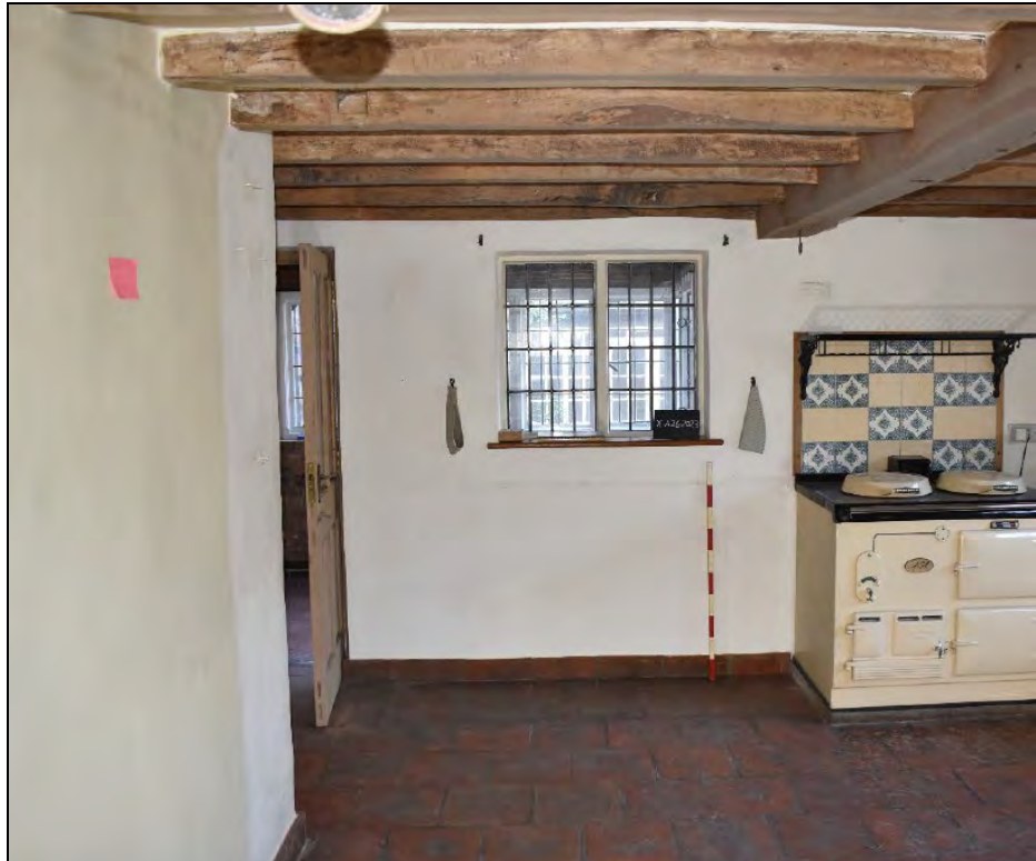
Plate 18: GF02 looking WNW (1.0m scale)
