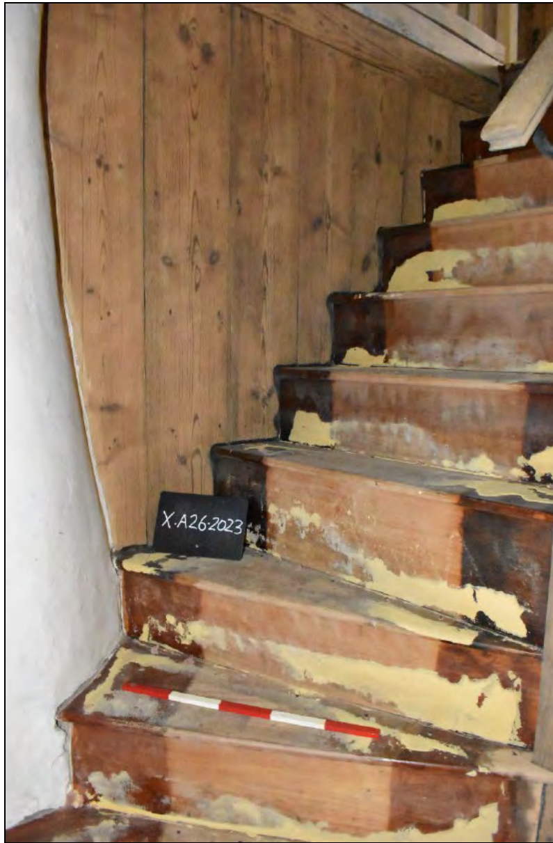
Plate 41: SF03 staircase looking WSW (50cm scale)
