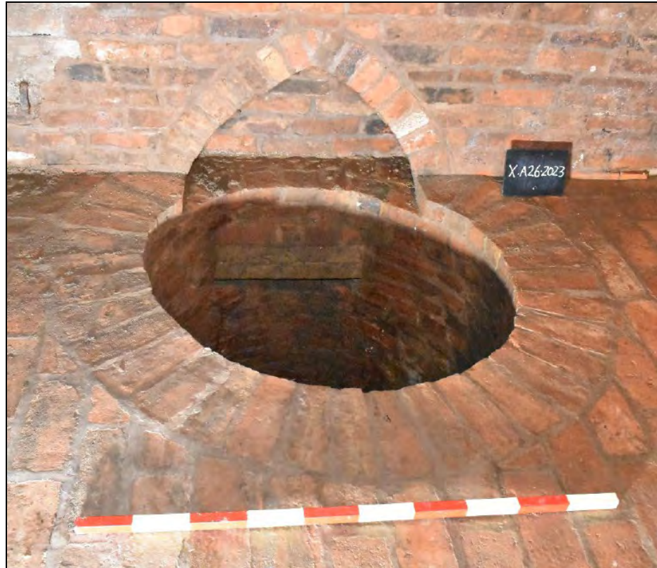
Plate 15: C01 well and relieving arch detail looking WNW (1.0m scale)
