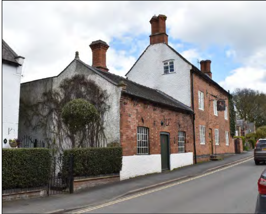
Plate 1: General view of Buildings A and B looking NE
