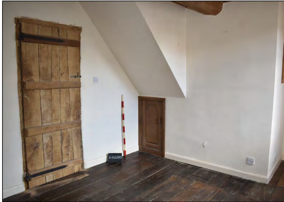
Plate 37: FF04 looking ENE (1.0m scale)
