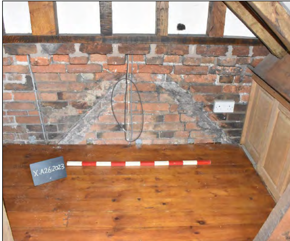
Plate 44: SF01 former gable scar looking SSW (1.0m scale)
