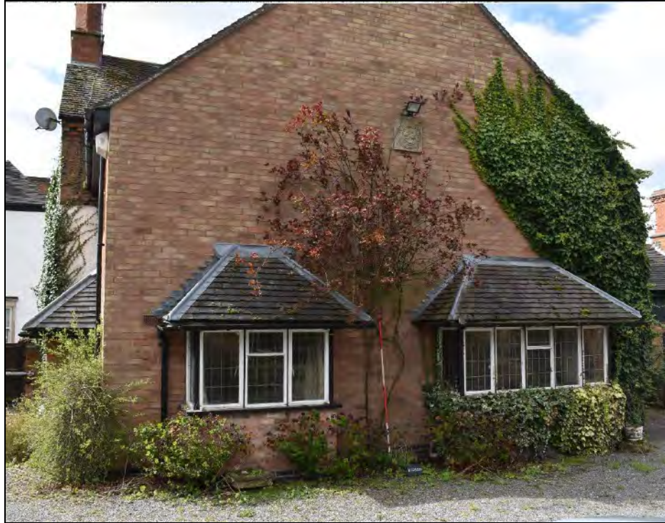
Plate 5: North elevation looking SSW (2.0m scale)
