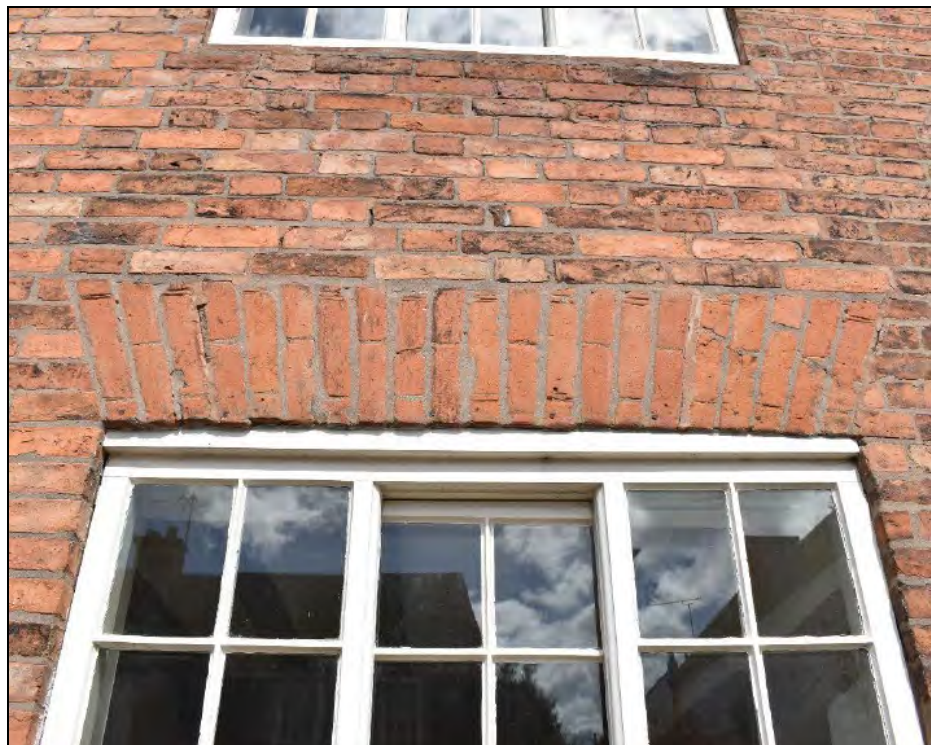
Plate 10: South elevation typical brick voussoir window head looking north
