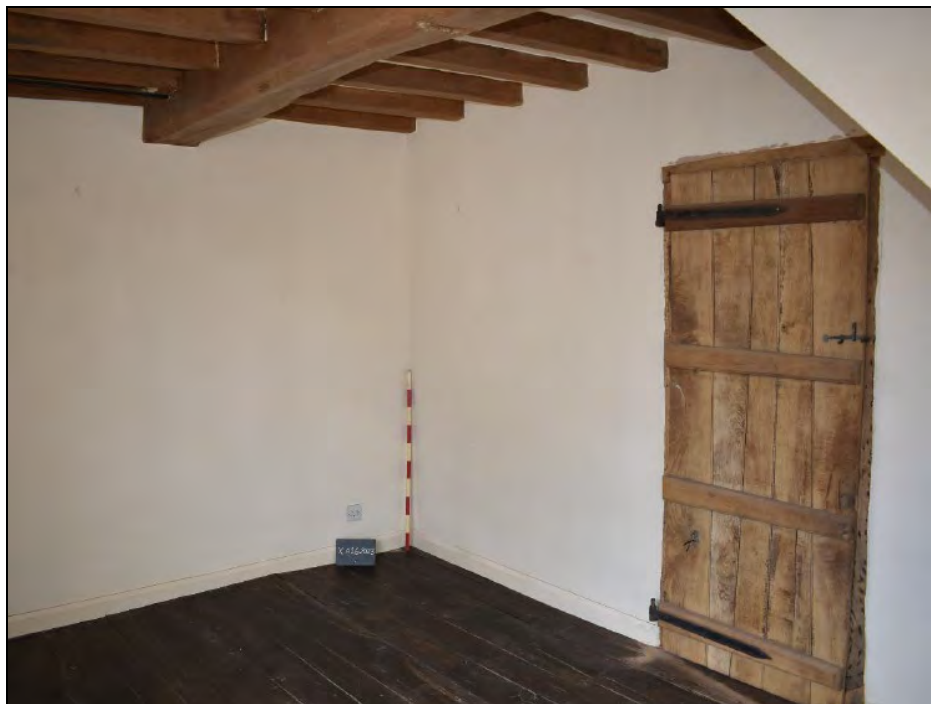
Plate 38: FF04 looking NW (1.0m scale)
