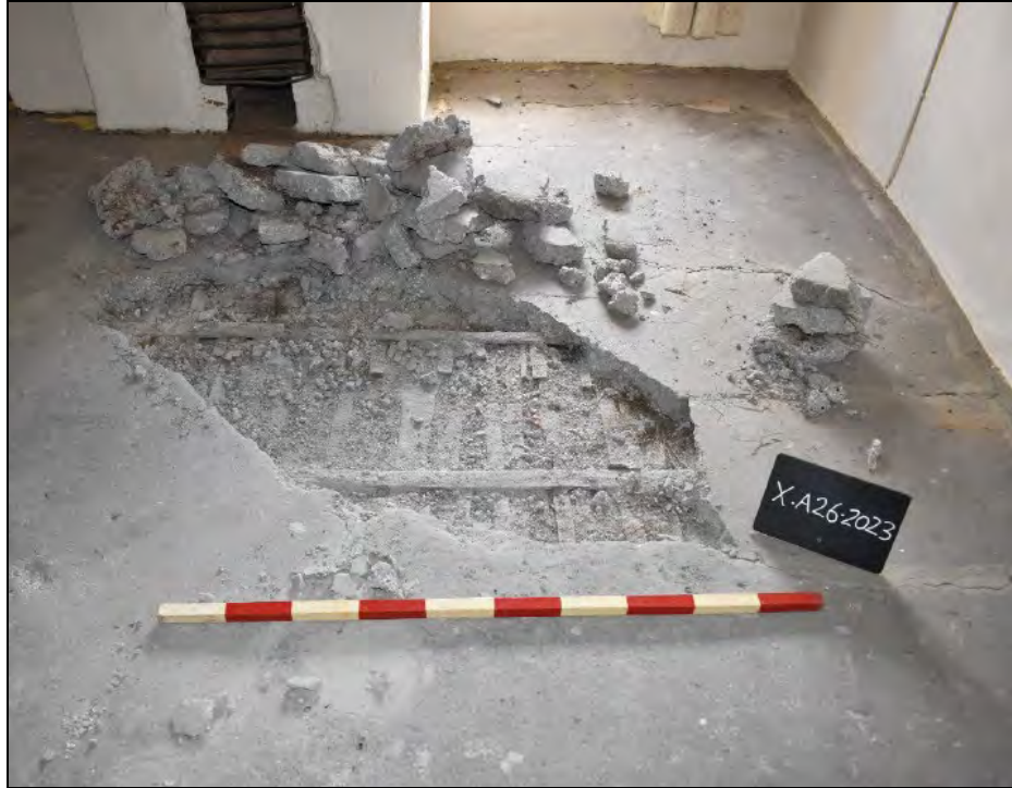
Plate 49: SF04 exposed lathe and screed floor looking ESE (1.0m scale)
