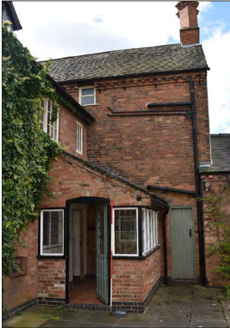
Plate 4: Porch GF01 looking south (2.0m scale)
