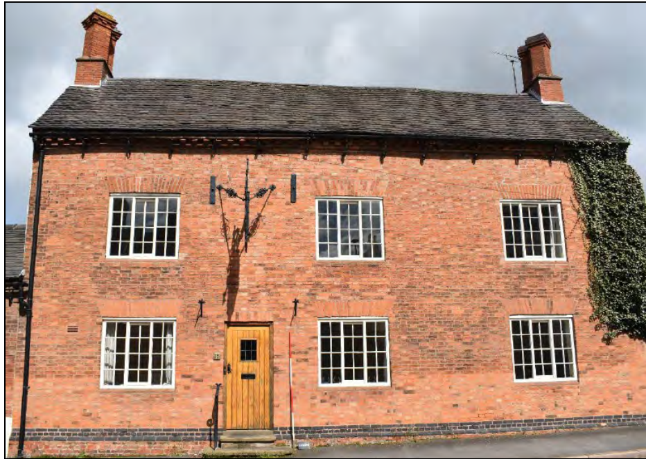
Plate 3: South elevation looking north (2.0m scale)
