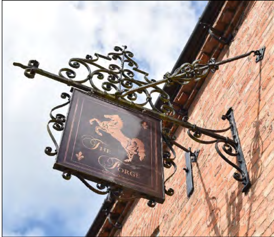
Plate 11: South elevation decorative cast-iron bracket and signage above main entrance
