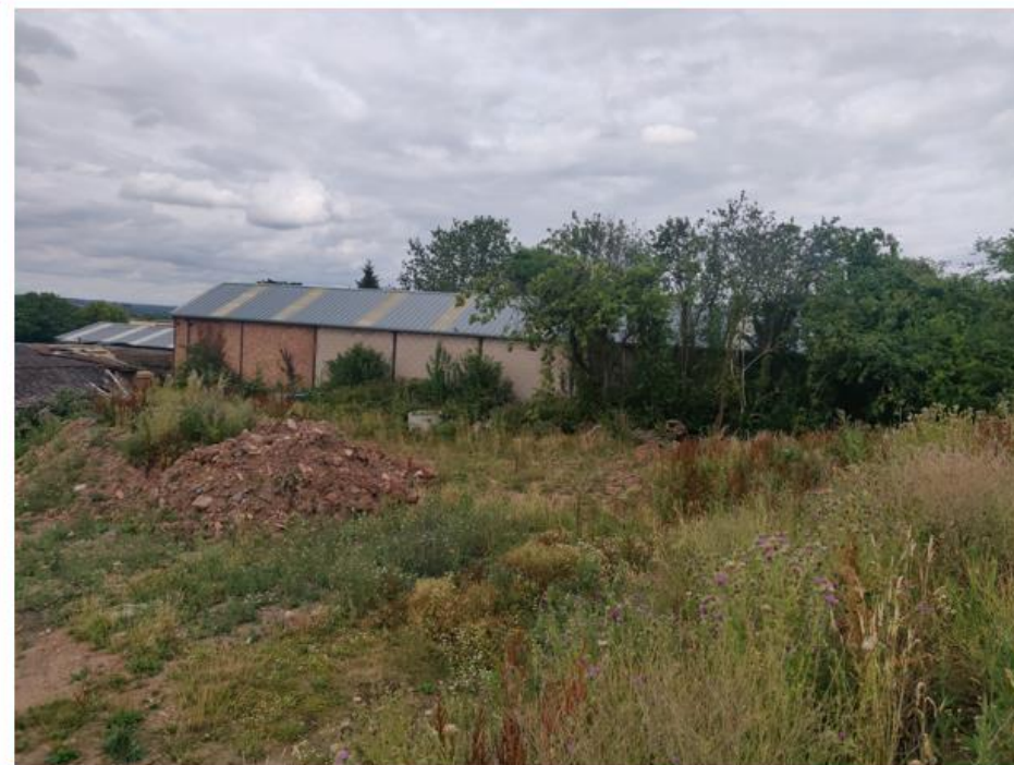
Photo No.14: Facing east towards the eastern extent of site showing further heaps and vegetated heaps
