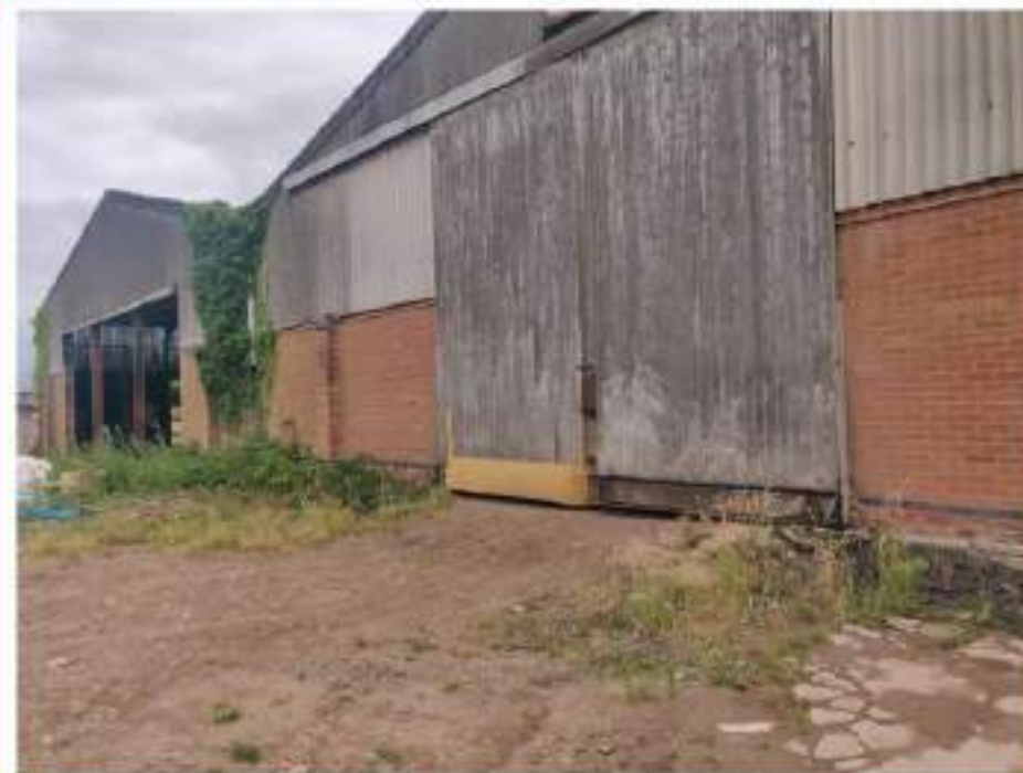
Photo No.6: Facing SE showing front (northern) faces of barns and PACM-cladding
