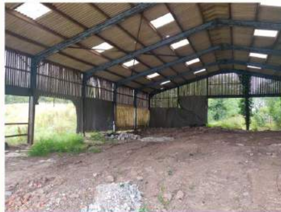
Photo No.10: facing south inside the eastern barn adjoined to that in the far west of site
