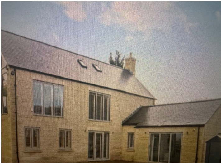
Timber windows and doors finished in Hardwick White
