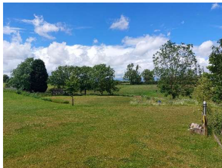
Existing balancing pond
