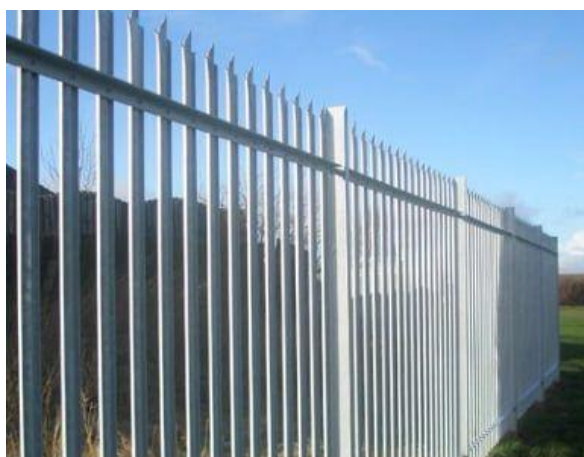
example of new galvanised palisade fencing, to match existing
