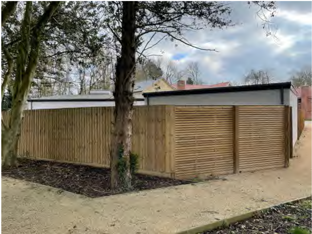
Existing public footpath showing existing rear garage/fencing finish on boundary
