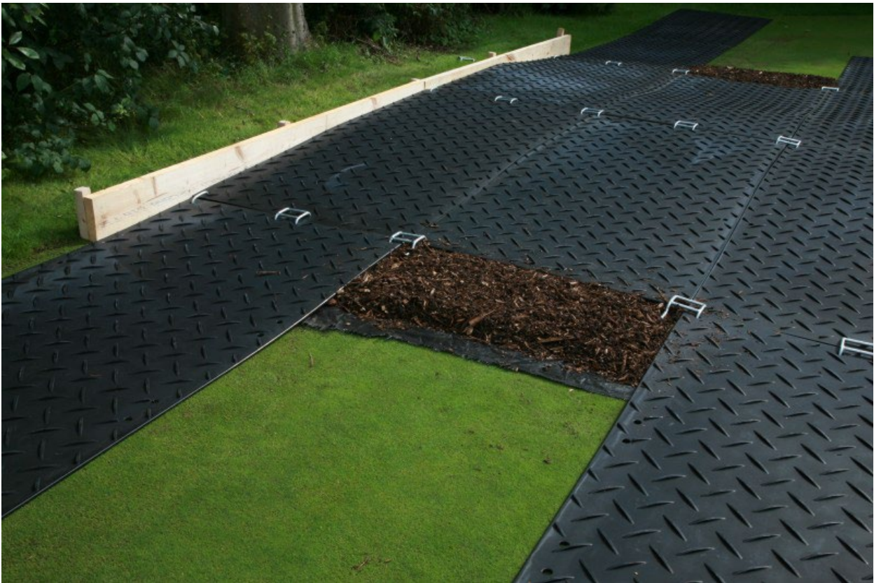
Image 1 – Ground-Guards temporary tree root protection - example
