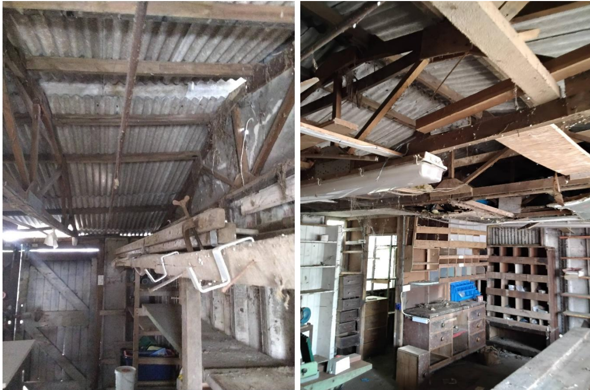
Photos 7 + 8. Internal structure of the garage building.
