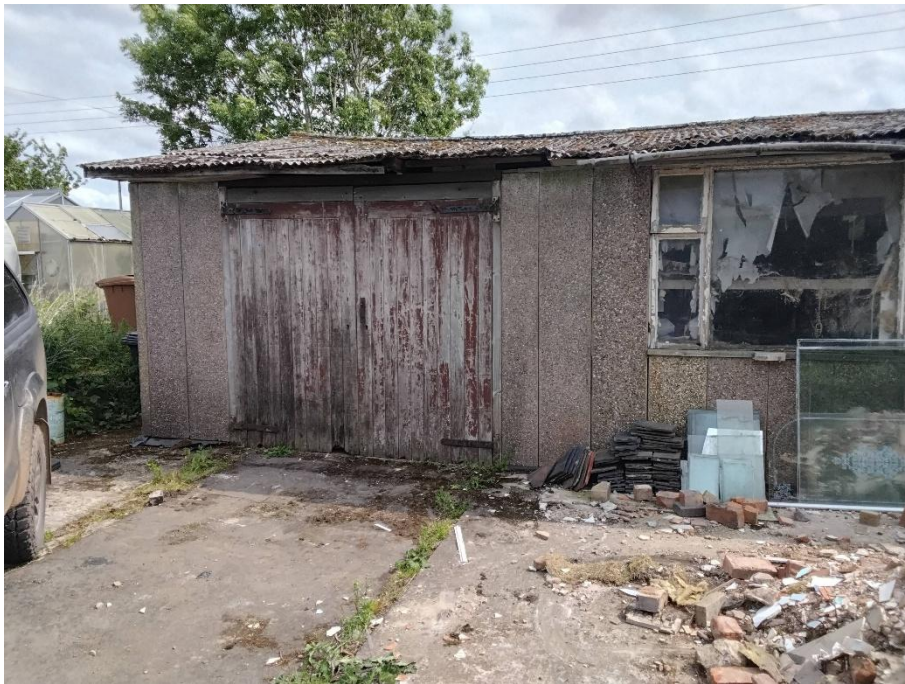
Photo 6. single-storey garage building present at the western end of the Site/
