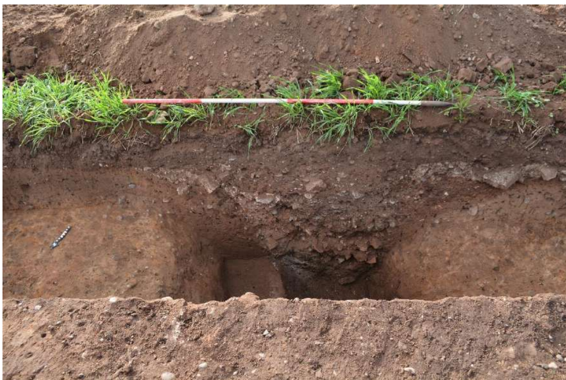
Plate 21 Trench 89, N facing section showing wall foundation cut [233] and robber cut [239] (x1 2m scale)
