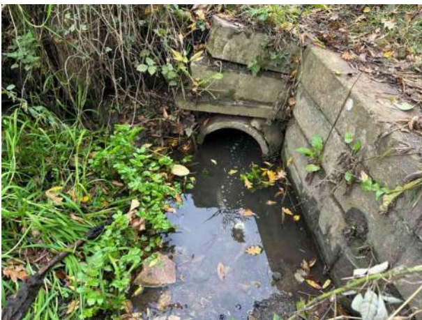
Outfall from SW1
