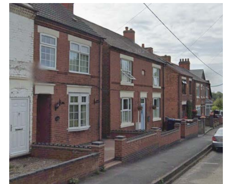
Low brick walls commonly define frontages.
