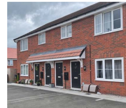
More recent interpretation of terraced housing with shared mono pitch door canopy.
