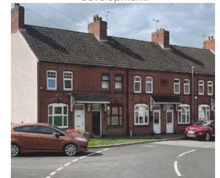
Slightly arched windows are a common feature in older properties.
