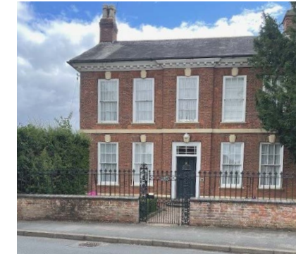
Historic, prominent buildings with brick, soffit and lintel detailing.
