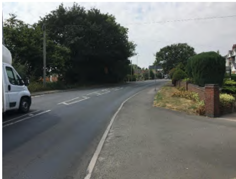
Photograph 1: Footways on Sapcote Road (west of Aston Flamville Road)
