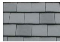
Grey interlocked roof tiles
