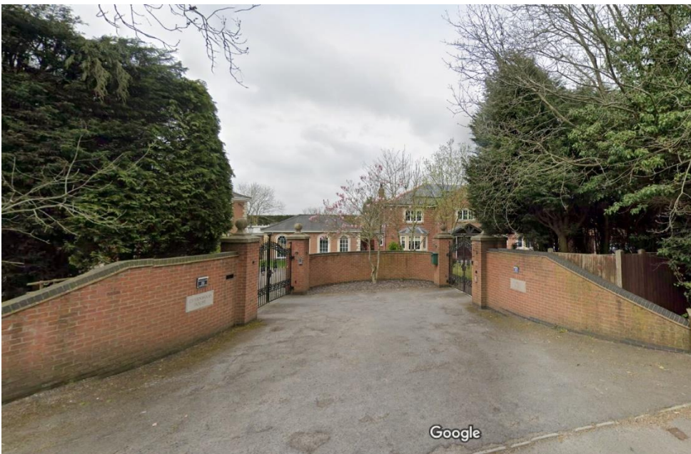
Charnwood House and Forest House. Large, mock Georgian style houses opposite the site. Red brick with stone detailing and grey roof tiles. Charnwood House (to the left) has mock Georgian sash windows whilst Forest House has modern proportioned casement windows.
