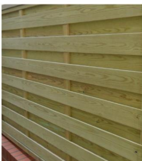
— New 1.8m timber hit and miss fencing
