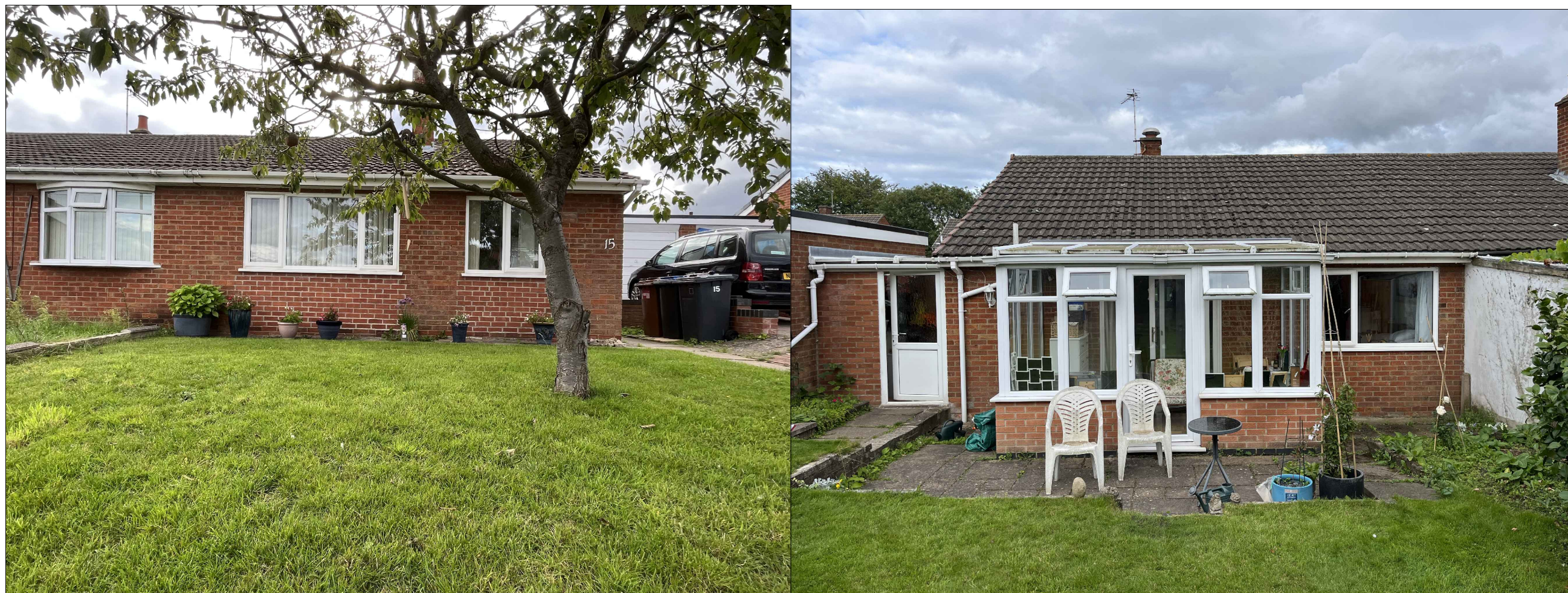
EXISTING SITE PHOTOGRAPHS - front elevation (L) and rear elevation (R)
