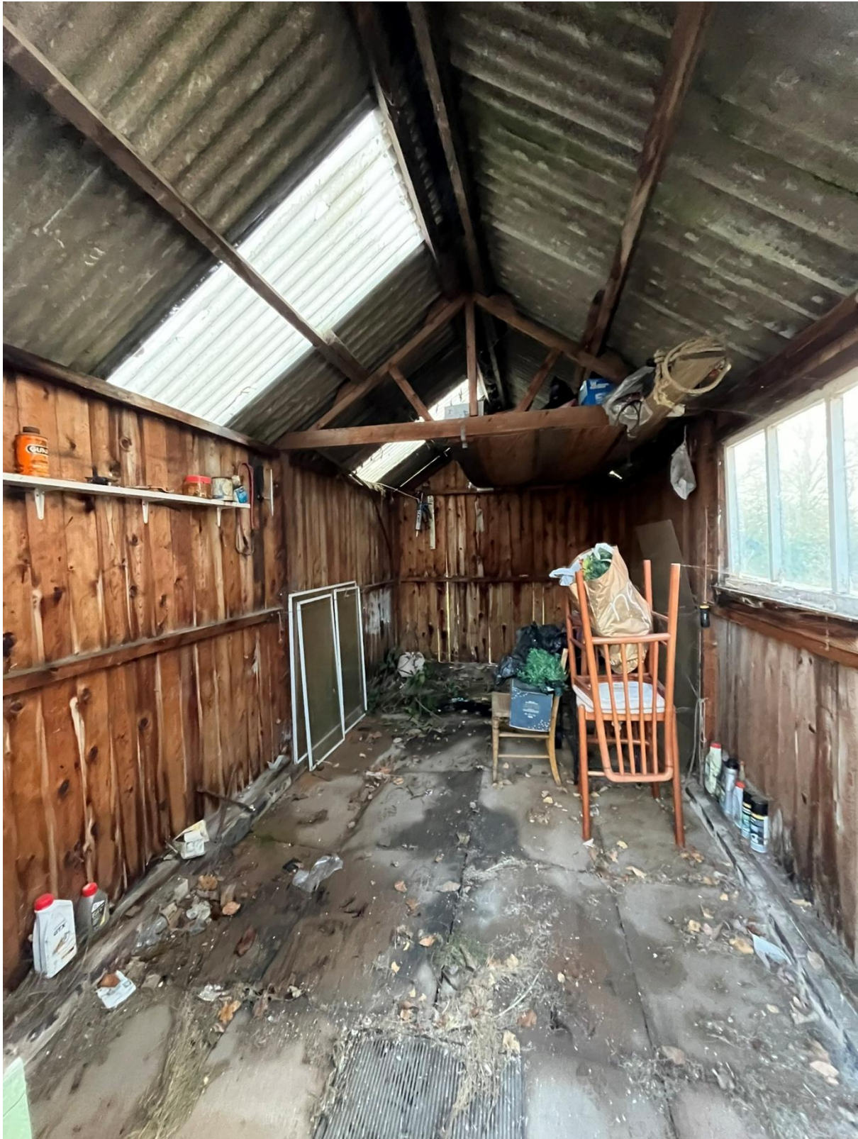
Photograph 8: The internal structure of the timber garage to the north-west of the site, showing the unsuitable internal fabric of the timber buildings.
