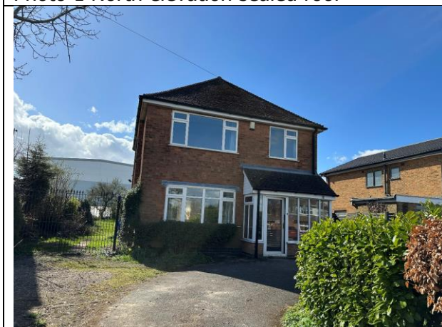
Photo 3 Sealed roof north east elevation
