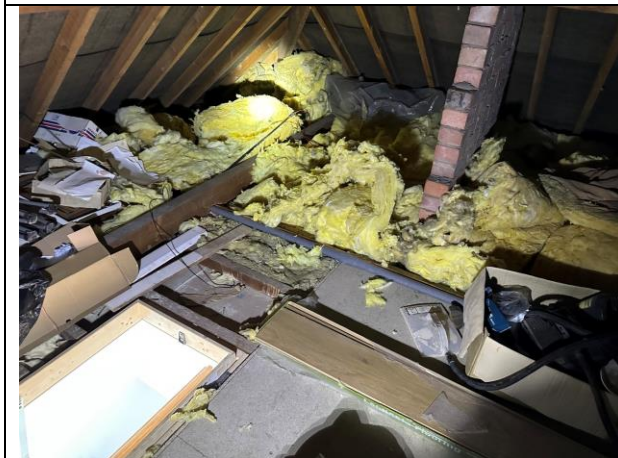
Photo 7 Clean loft floor
