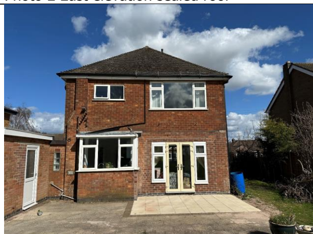
Photo 4 Sealed roof south west elevation
