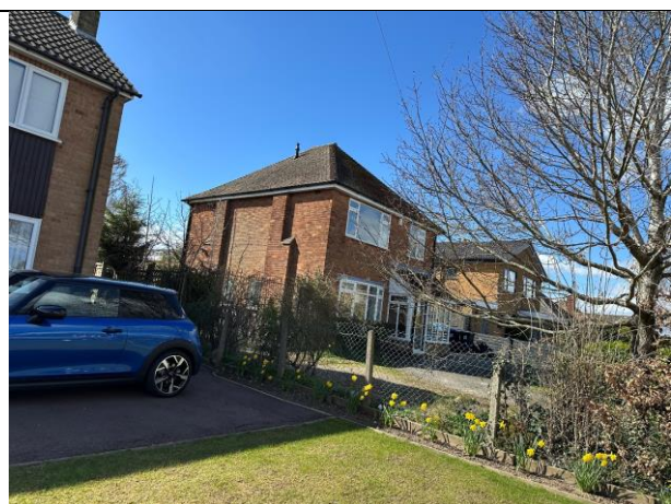
Photo 2 East elevation sealed roof
