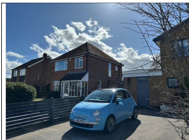
Photo 1 North elevation sealed roof
