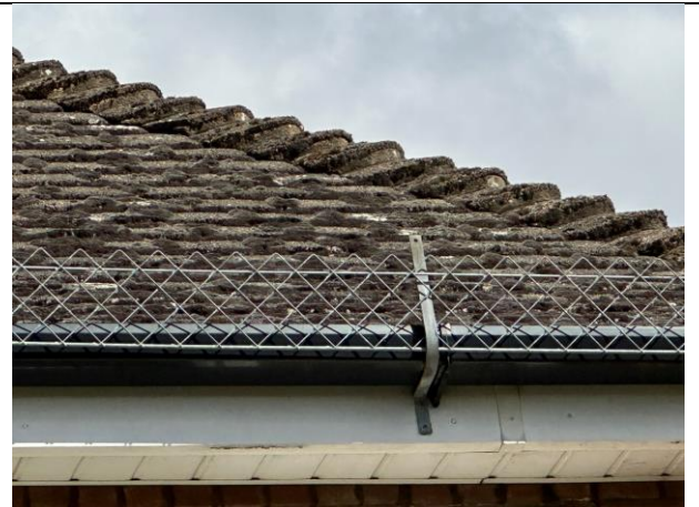
Photo 6 Sealed bonnet tiles
