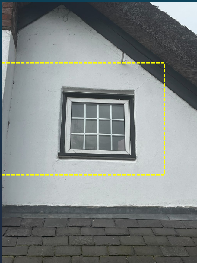
Window 16 Upper Bathroom
