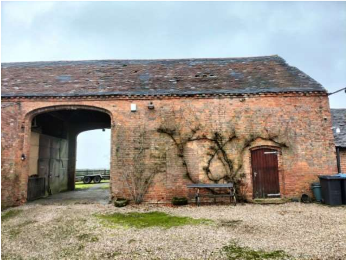
15. View north from near centre of the quadrangle, towards storage barn along the northern side of the quadrangle.
