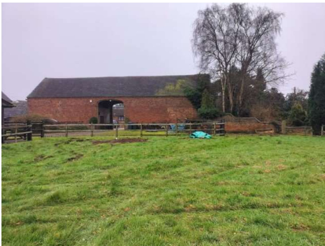
1. View south across the site from near the northern boundary towards the northern elevation of the barn on the northern side of the quadrangle.
