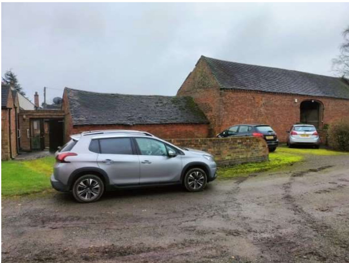
26. View south towards the north-eastern corner (external) of the quadrangle buildings. Access archway on right hand side to quadrangle courtyard is visible.
