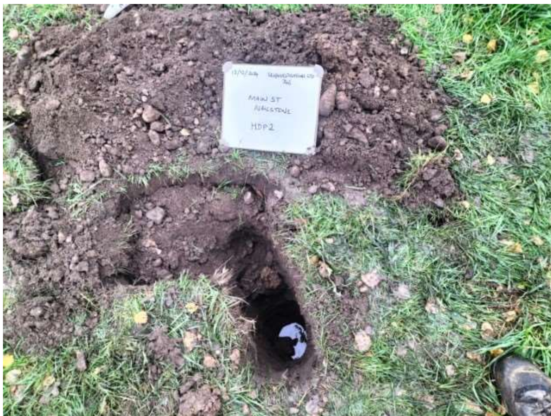
Hand dug pit HDP2.
