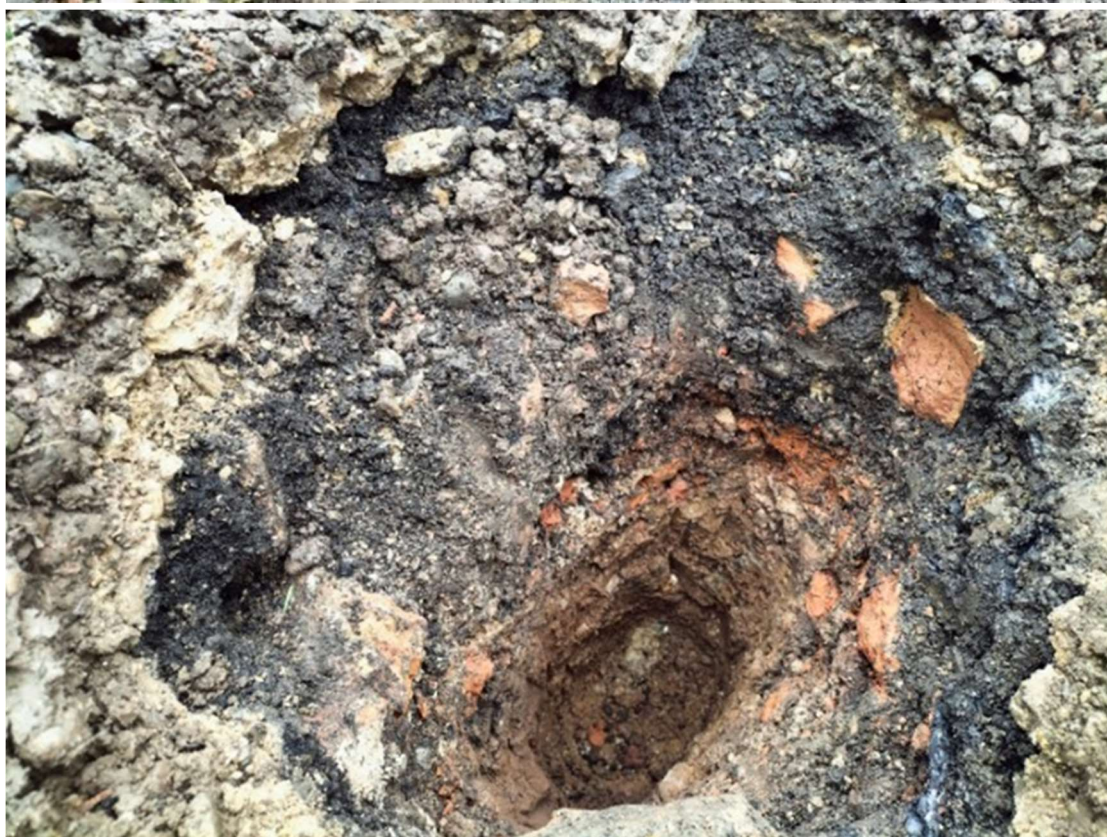
Hand dug pit HDP2.
