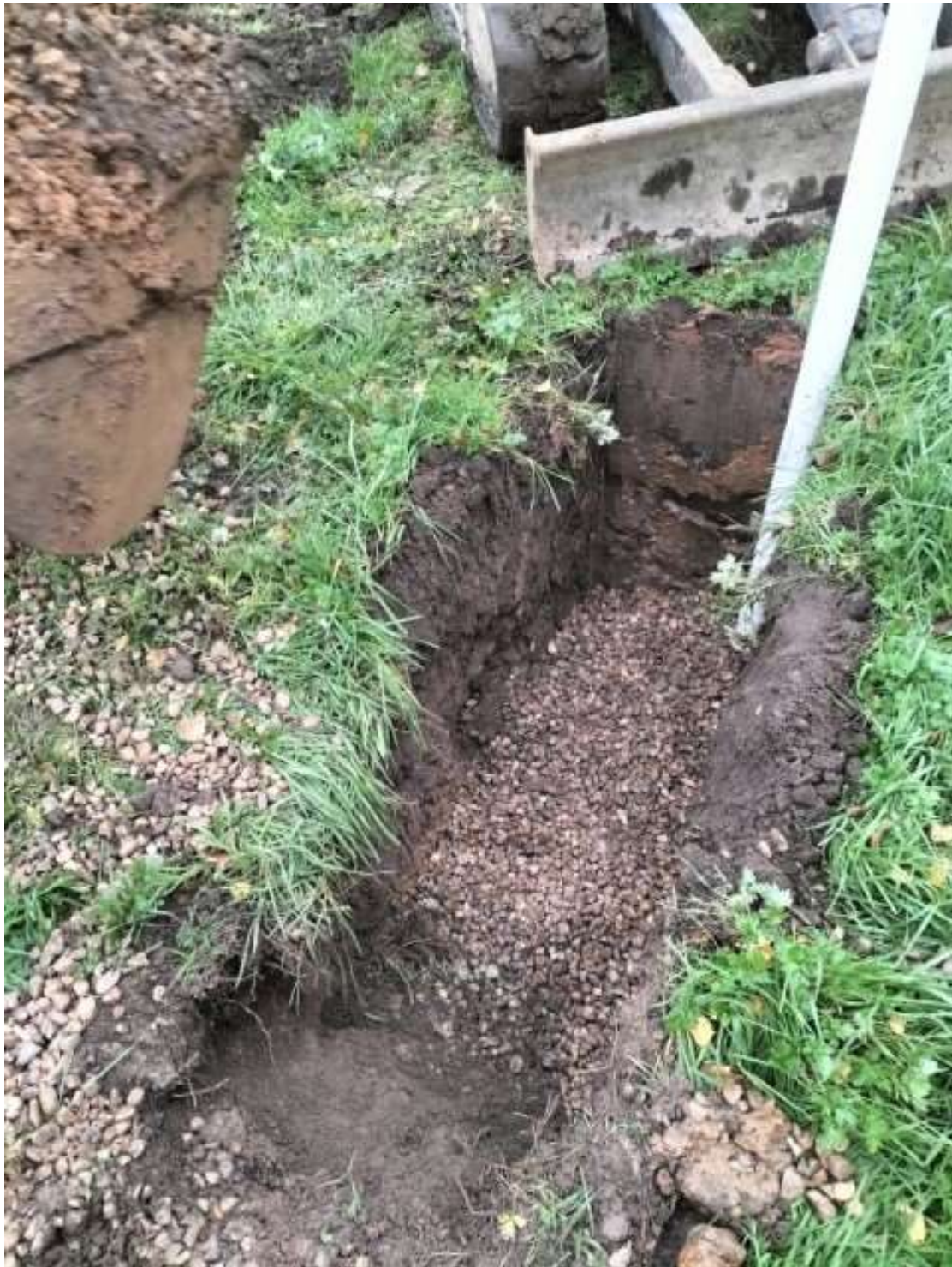
Soakaway test pit TP SA1, after placement of groundwater monitoring standpipe and single sized gravel.
