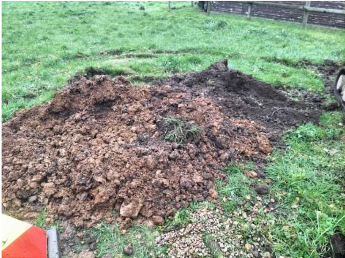
Excavation spoil from TP SA1.
