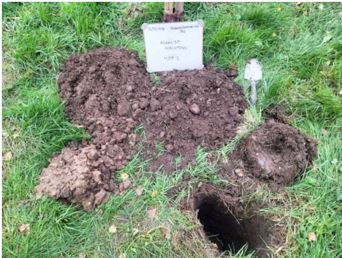
Hand dug pit HDP1.
