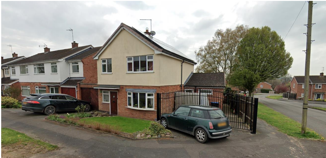
Streetview of a gable fronted dwelling, adjacent to gable ended houses, on a nearby corner plot on a junction with Danes Hill
