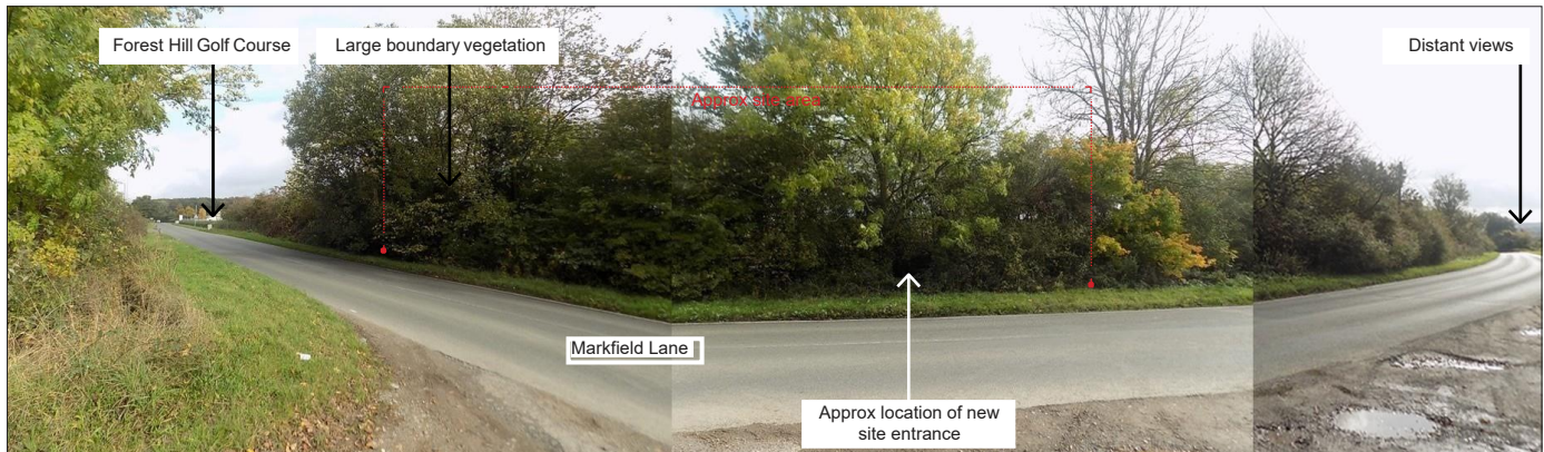
02 - View east from public footpath of Markfield Lane.
