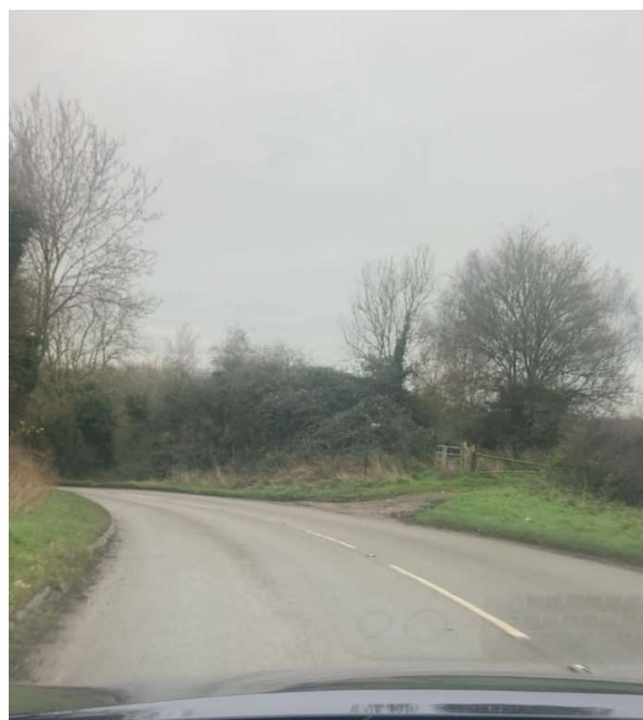
View looking north-east: similar issues with alignment and cresting
