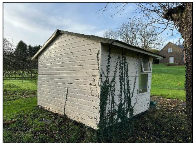
Photograph 47: Rear and side (north) view.
