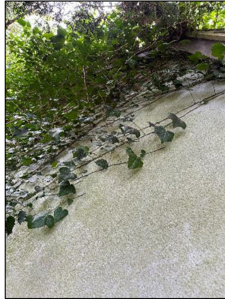
Photograph 45: Rear view of B1 with ivy-clad walls.
