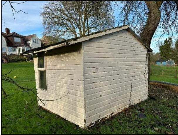
Photograph 48: Rear and side (south) view.
