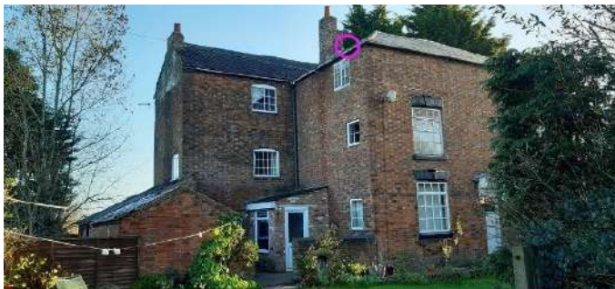
Photograph 2: B4a eastern elevation- bat roost location.
