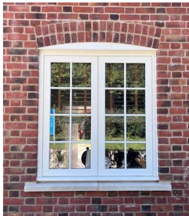
Window Arrangement – SW Timber Windows / Constituted Stone Cill / Brick Header
