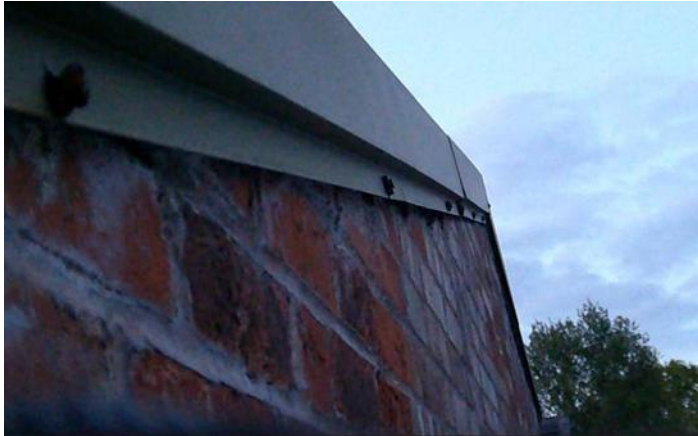
Photo 1. Metal bargeboards at B1 can be unbolted and removed by hand for inspection and replaced if signs of bats are discovered.
