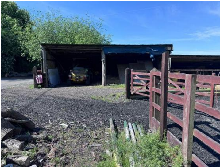
Photo 3. Facing southwest toward one section of B2. The semi-mature tree to be retained can be seen to the rear (left). This tree will require root protection during demolition and ground works if required. Should the tree require felling, it should be replaced with like for like at a ratio of 2:1.
