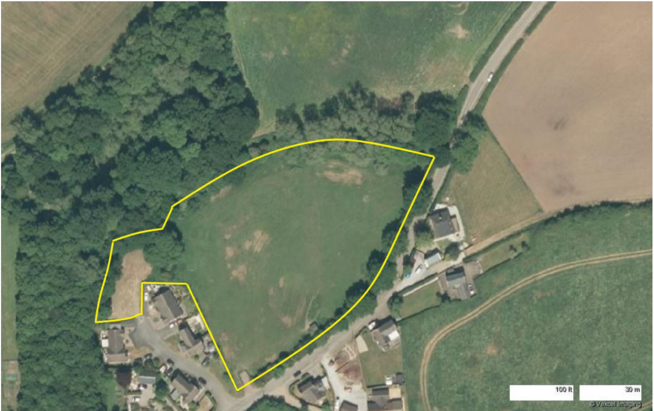
Figure 2: Site Contextual Aerial Photograph
