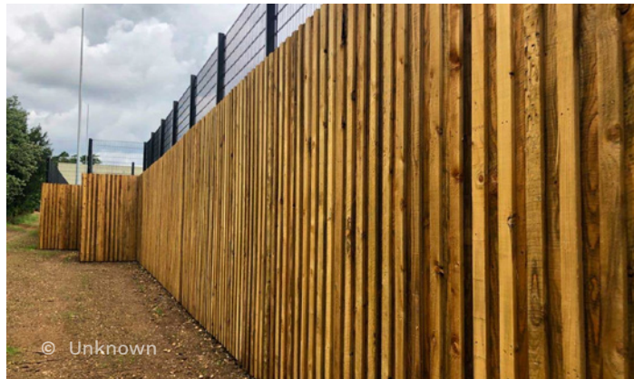
Closeboard fencing for screening of BOH Facilities
