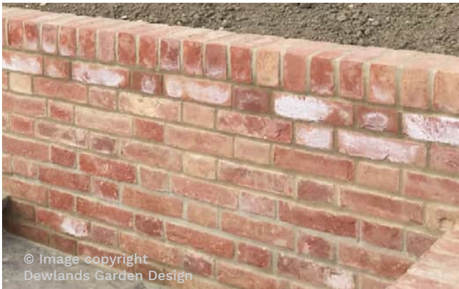
Textures – brick walls and seating to ‘Teaching Garden’
