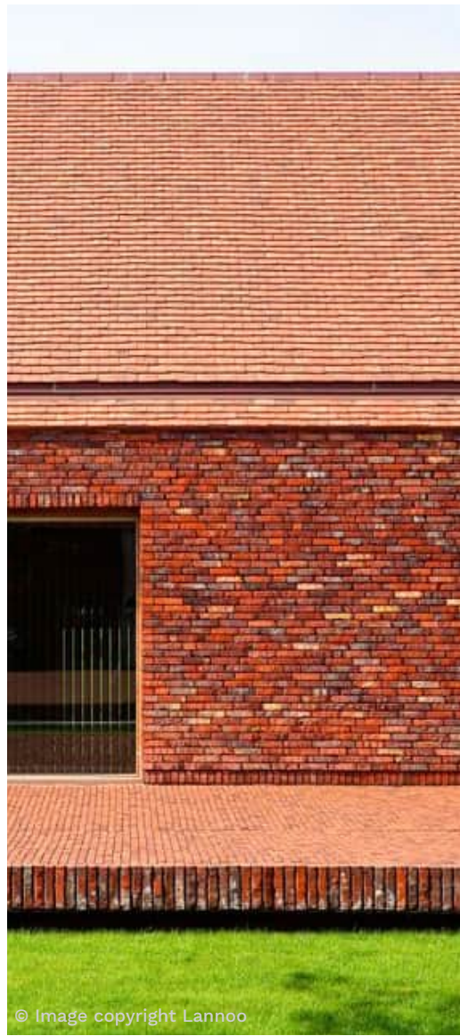
Farmhouse Renovation Buro II & Archi+I
