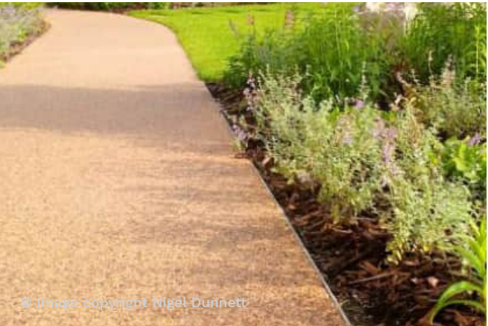
Surface – Porous resin bound gravel to pathways around the building and linking to the Zoo
