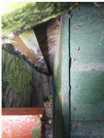
Plate 4.14: Side of shed West
