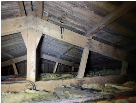
Plate 4.7: Loft with insulation
