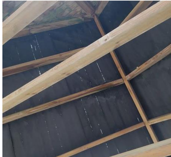
Plate 4.21: Inside of northern wooden porchway
