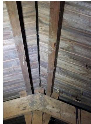
Plate 4.6: Tightly fitted wooden boards
