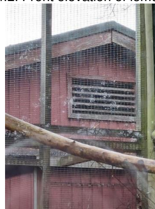
Plate 4.4: Air vent at rear of lemur house
