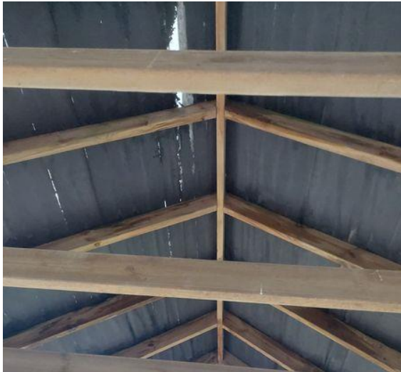
Plate 4.20: Inside of northern wooden porchway
