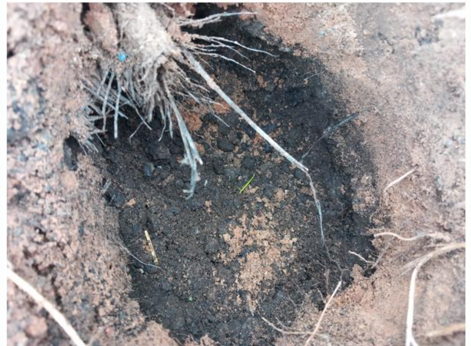
Photo No.2: IP01 pit sides and base showing ménage sand material atop membrane atop ashy subbase made ground
