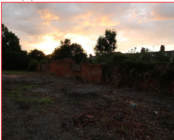
View of Northern Boundary wall – residencies beyond
