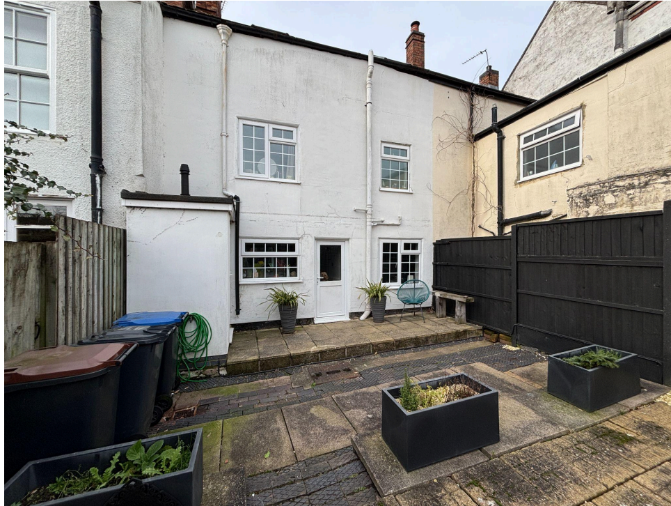
Existing rear aspect
