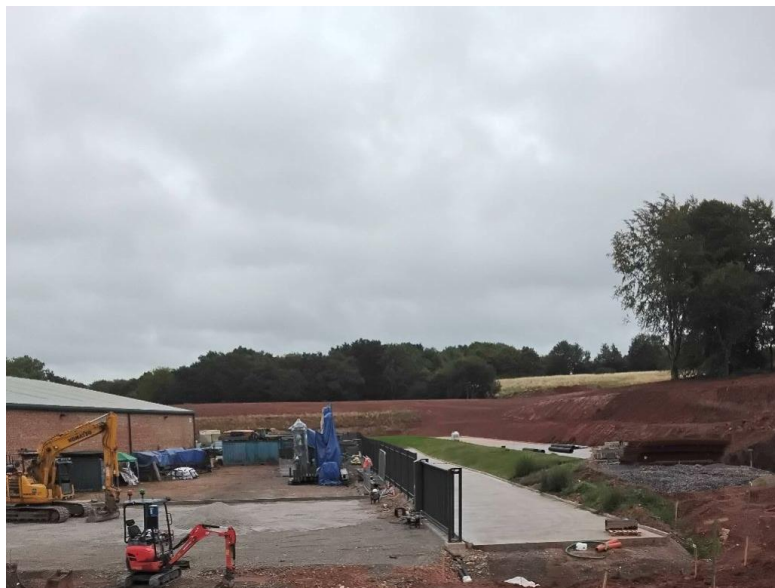
Figure 4. Unsealed surface at the south of the Site, with southern elevation of the existing building to the left of shot
