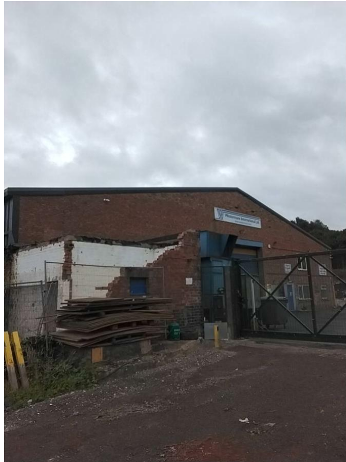
Figure 3. Main building at the Site (Northwest elevation)
