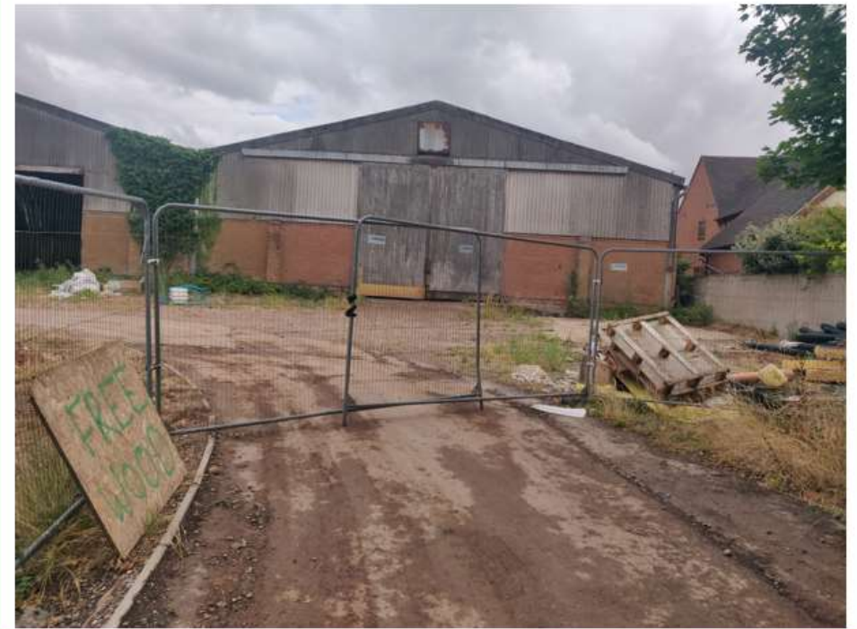
Photo No.2: Facing south from the site access showing the large barns forming the western extent of site
