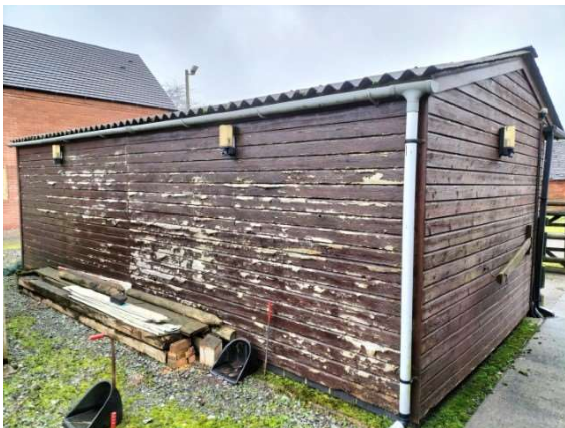
21. Western elevation of the wooden storage shed.
