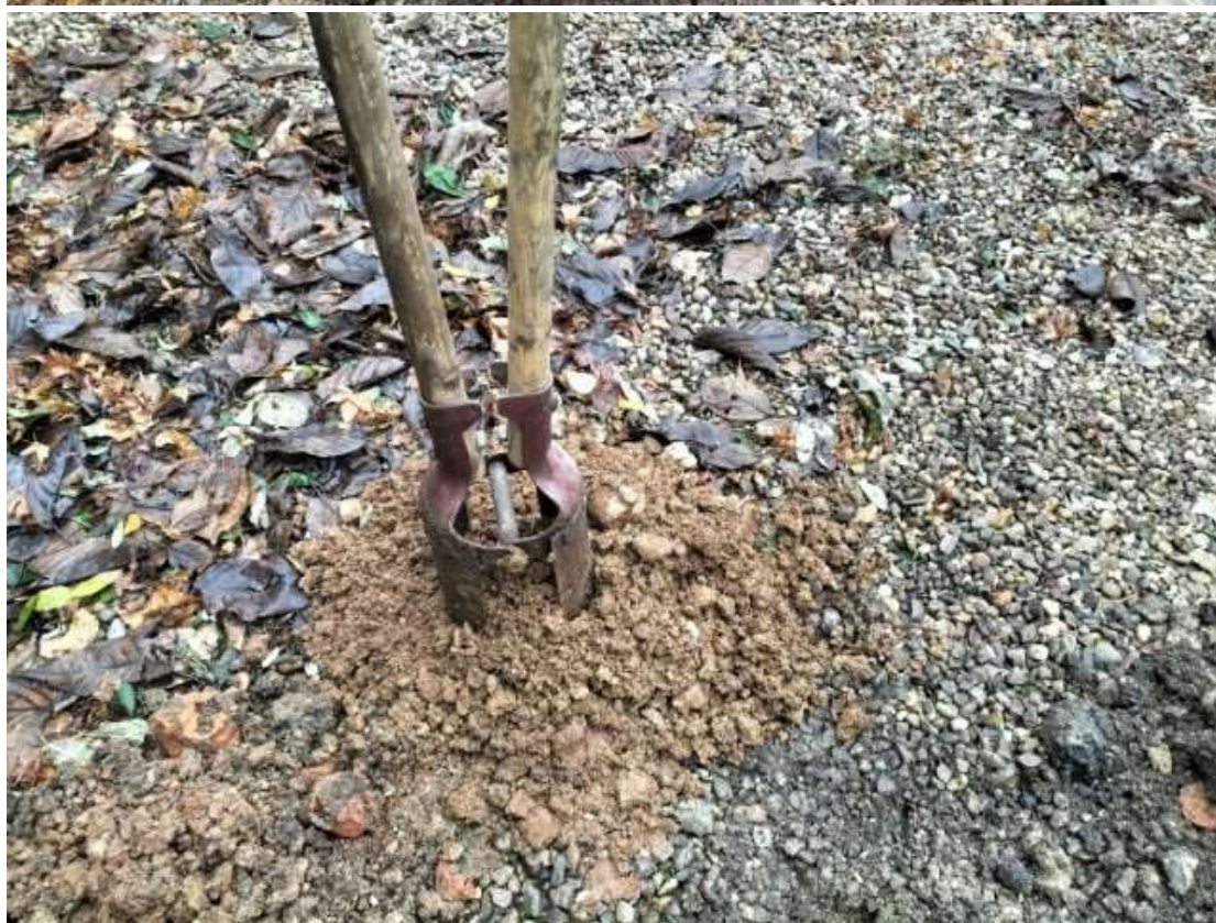
Hand dug pit HDP2, showing made ground excavation arisings above the natural sandy gravel below.
