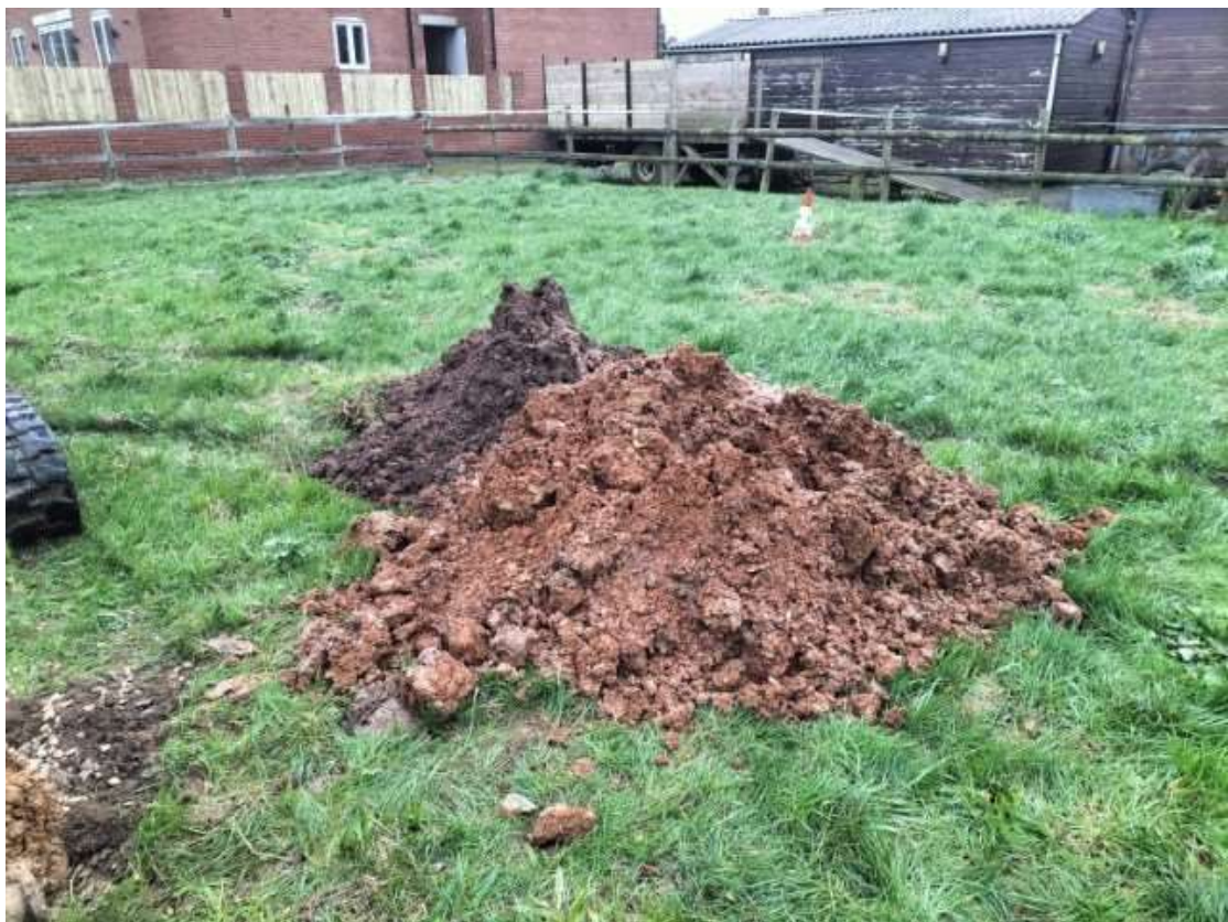
Excavation spoil from soakaway test pit TP SA2.
