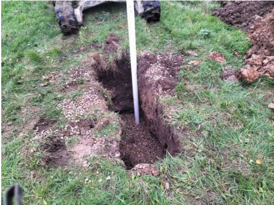
Soakaway trial pit TP SA2 after placement of groundwater monitoring standpipe and single sized gravel.
