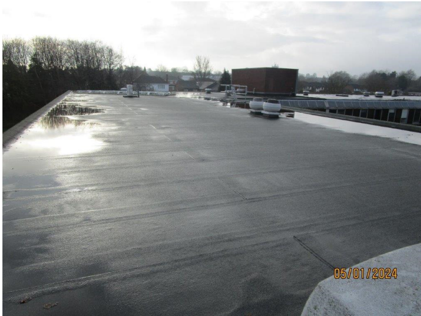
Roofing for replacement.
