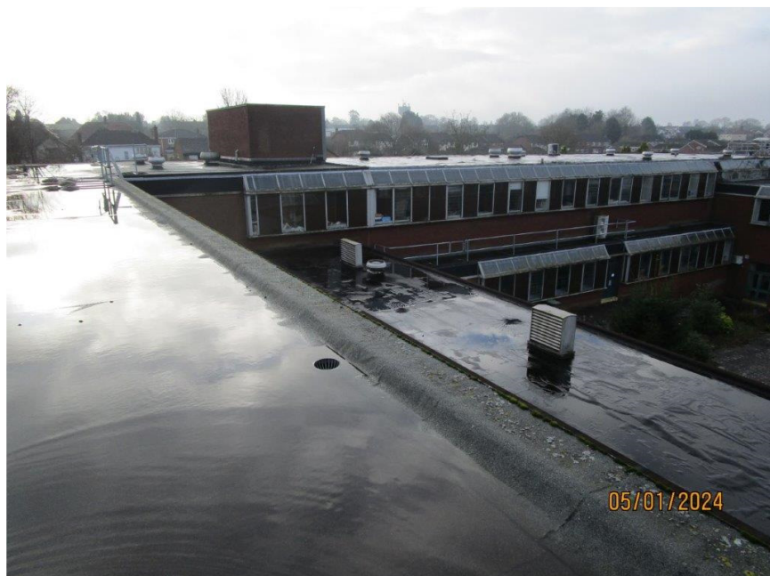
Roofing for replacement.
