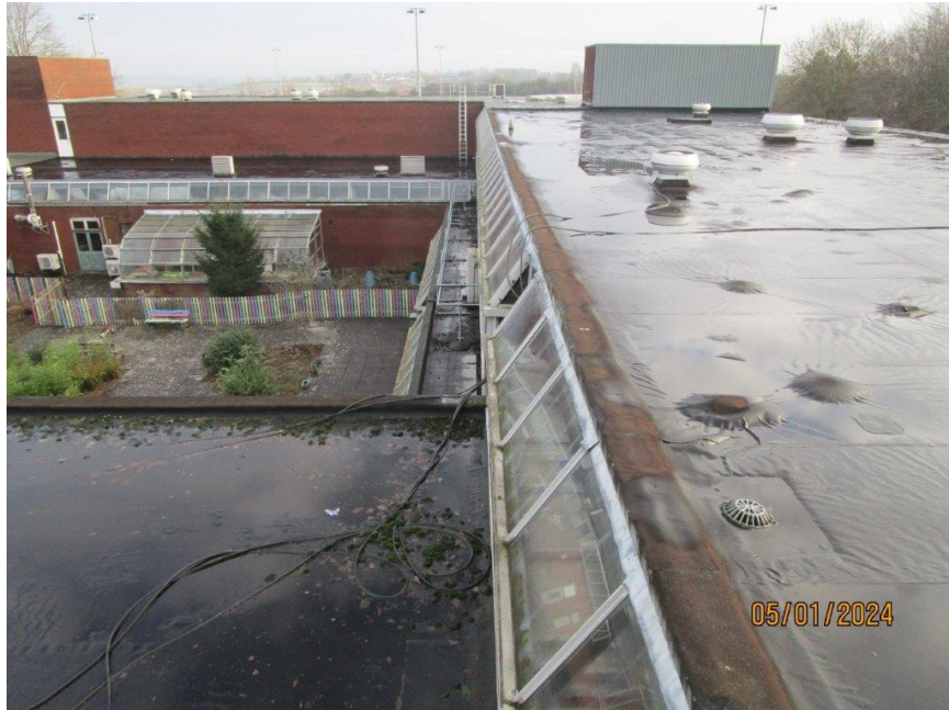
Roofing for replacement.
